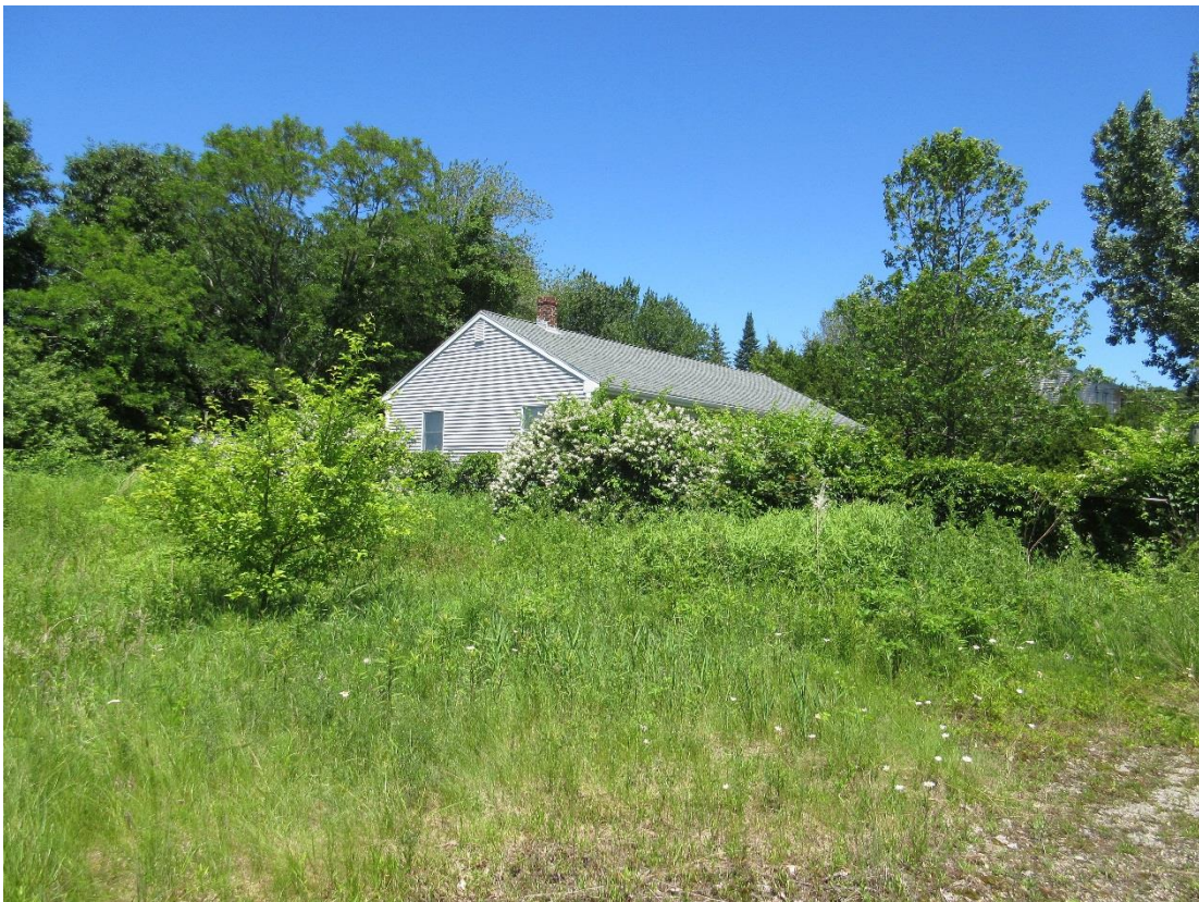
Photo 8: Adjacent residence off the northwest corner of the subject site.
