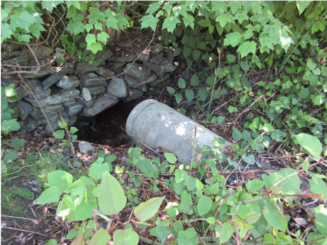
Photo 3: Culverted drainage ditch bisecting the center of the subject site.
