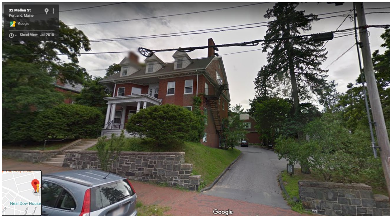
Figure 1: Main House facade
