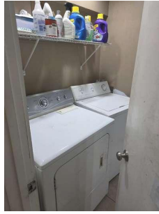
Unit 4 Laundry Utility
