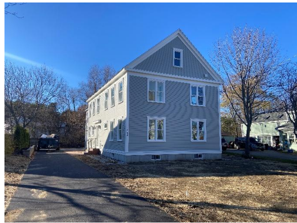
Figure 9: Recent Construction at 1164 Westbrook
