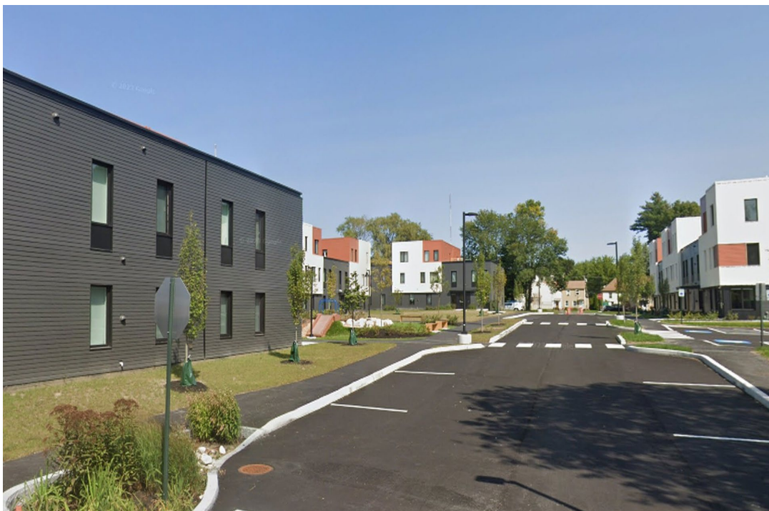
Front Street East: rebuilt affordable family housing in East Deering
