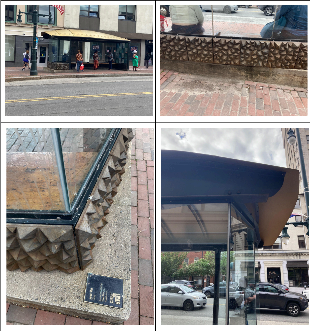
Figure 3 - Existing condition photos from May 28, 2026
