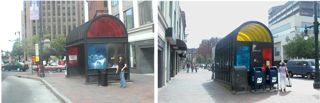
Figure 2: Former bus shelter prior to 2004 Jewel Box installation
