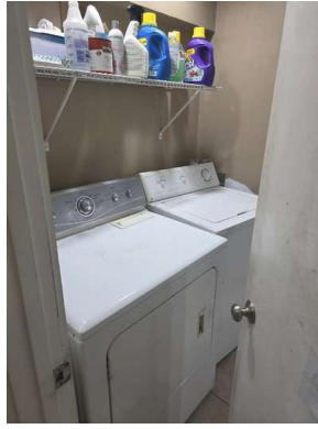
Unit 4 Laundry Utility
