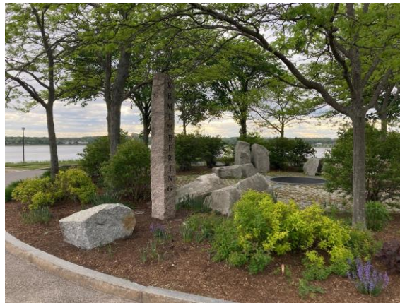
Image of repair to reset existing granite, May 2026
