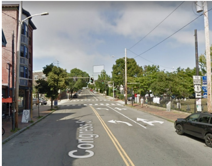
Figure 4: Lane striping at Congress Street at Washington Avenue
