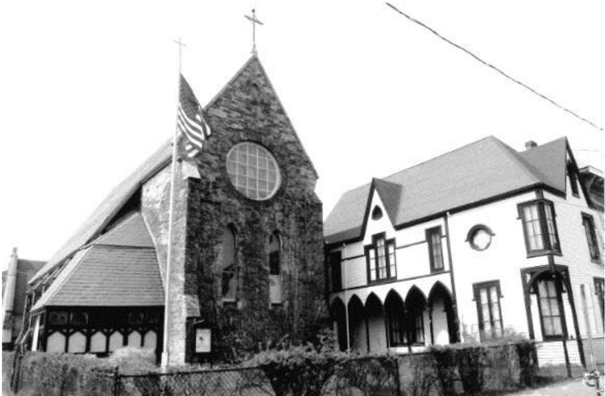
Figure 3: 1993 Photo showing the rectory with the altered porch and vinyl siding.
