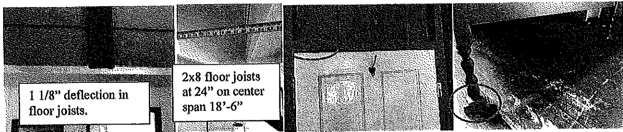
Photograph 2 : Second floor framing. Joists are under-sized causing severe sag in second floor. Note typical second floor door and 2 1/4" block required to level bed.
