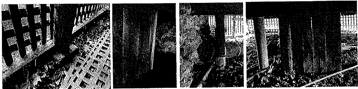
Photograph 3 : Structural deficiencies. There is no foundation, tree posts on blocks and support walls in direct contact with the ground make up most of the building support.
