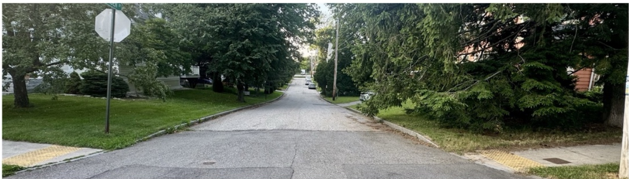
MISSING SIDEWALKS — BOTH SIDES OF LINDEN STREET
