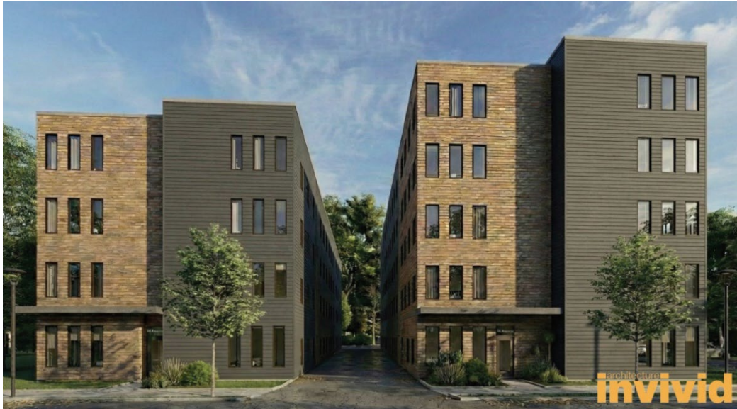
Streetview from Ashmont Street.
