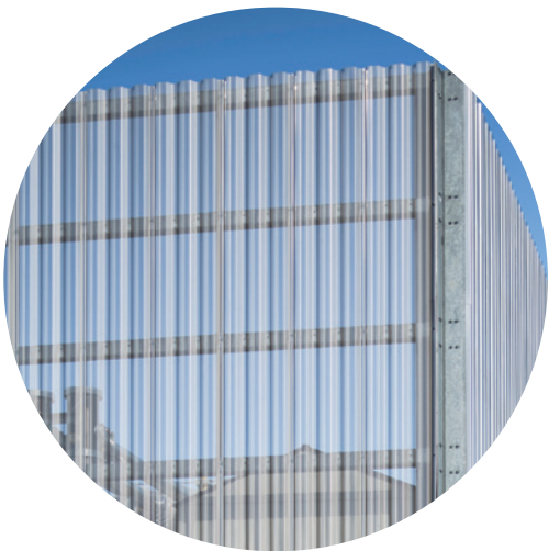
CORRUGATED PERFORATED SCREEN SCREENING WILL BE PROVIDED AROUND MECHANICAL UNITS ON BUILDING 14.
