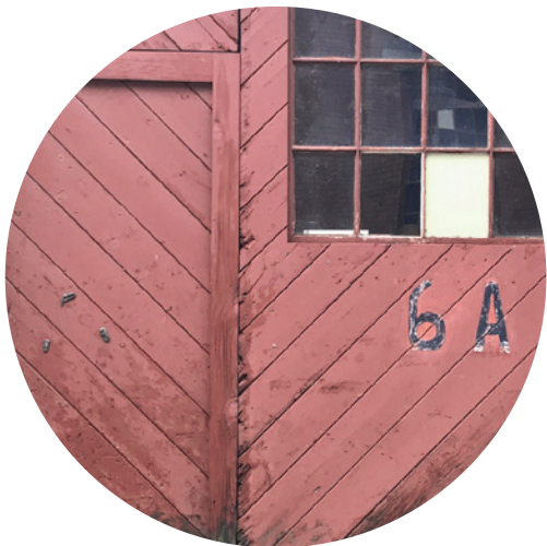
PAINTED T&G SIDING T&G SIDING TAKES A CUE FROM THE INFILL SIDING FOUND THROUGHOUT THE SITE.
