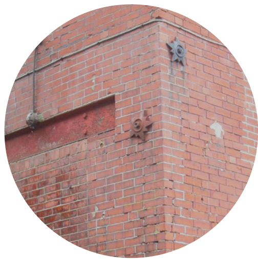
RESTORED BRICK Masonry remaining at Building 24, Buidling 15, and Building 16 will be repaired.
