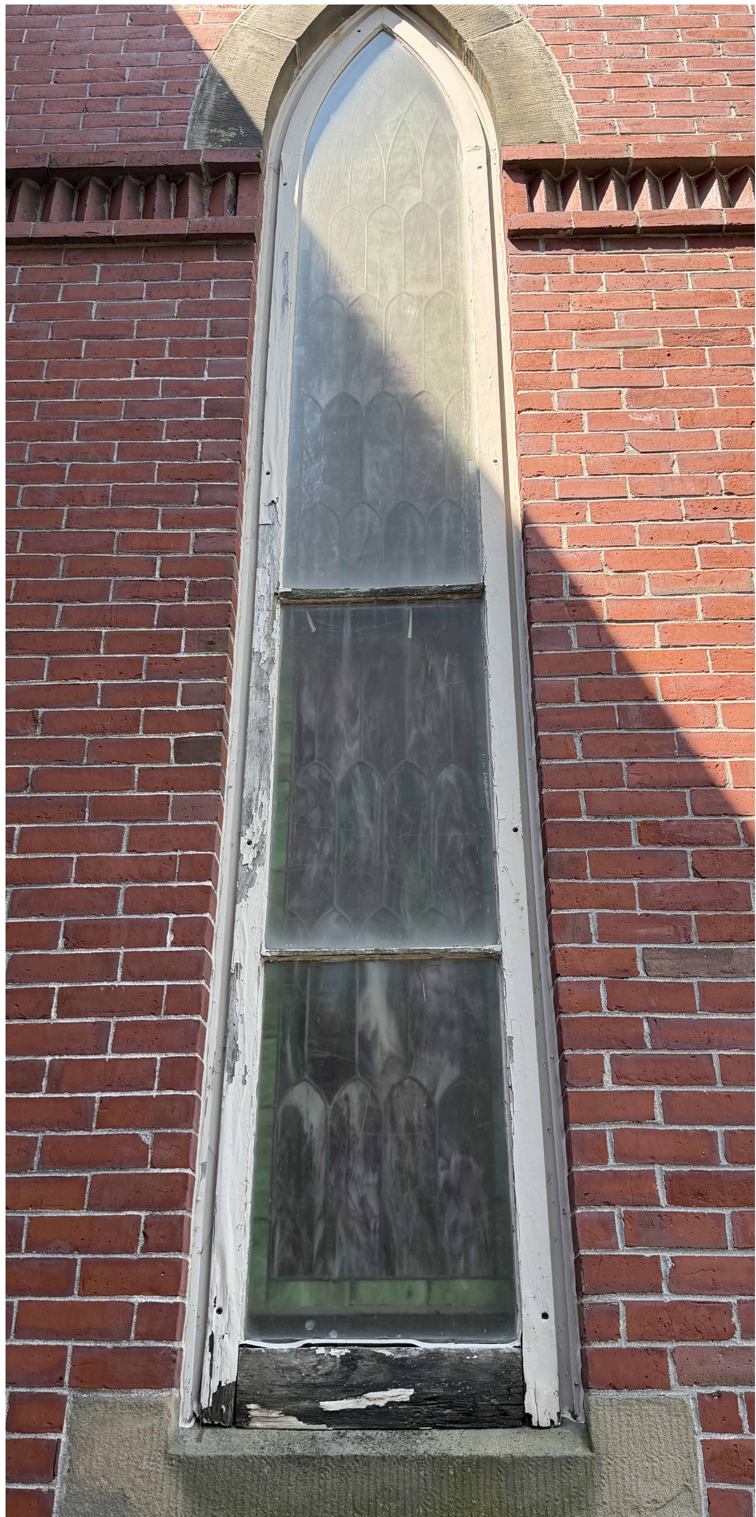
TYPICAL EXISTING EXTERIOR WINDOW TRIM | 4
