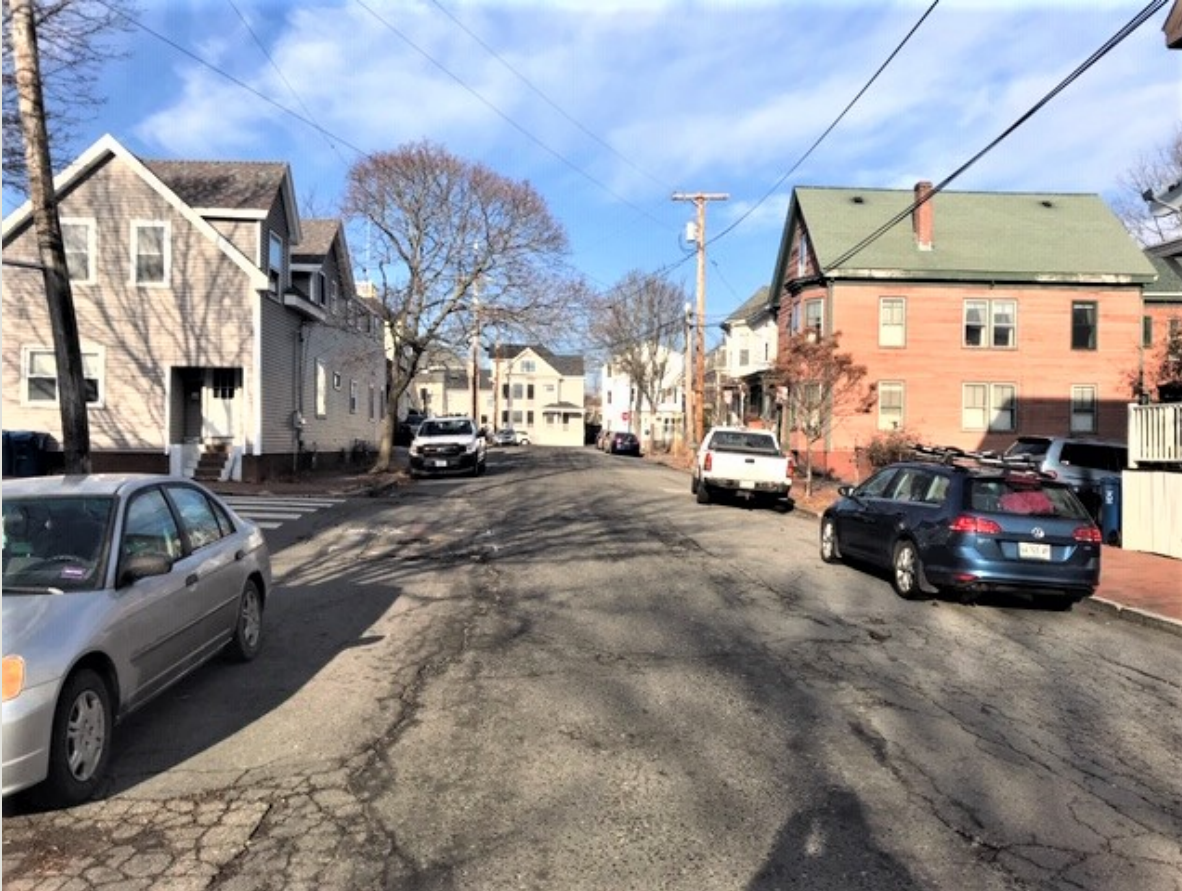
Munjoy Street – PCI = 39; ranked Very Poor Rehabilitation treatment recommendation
