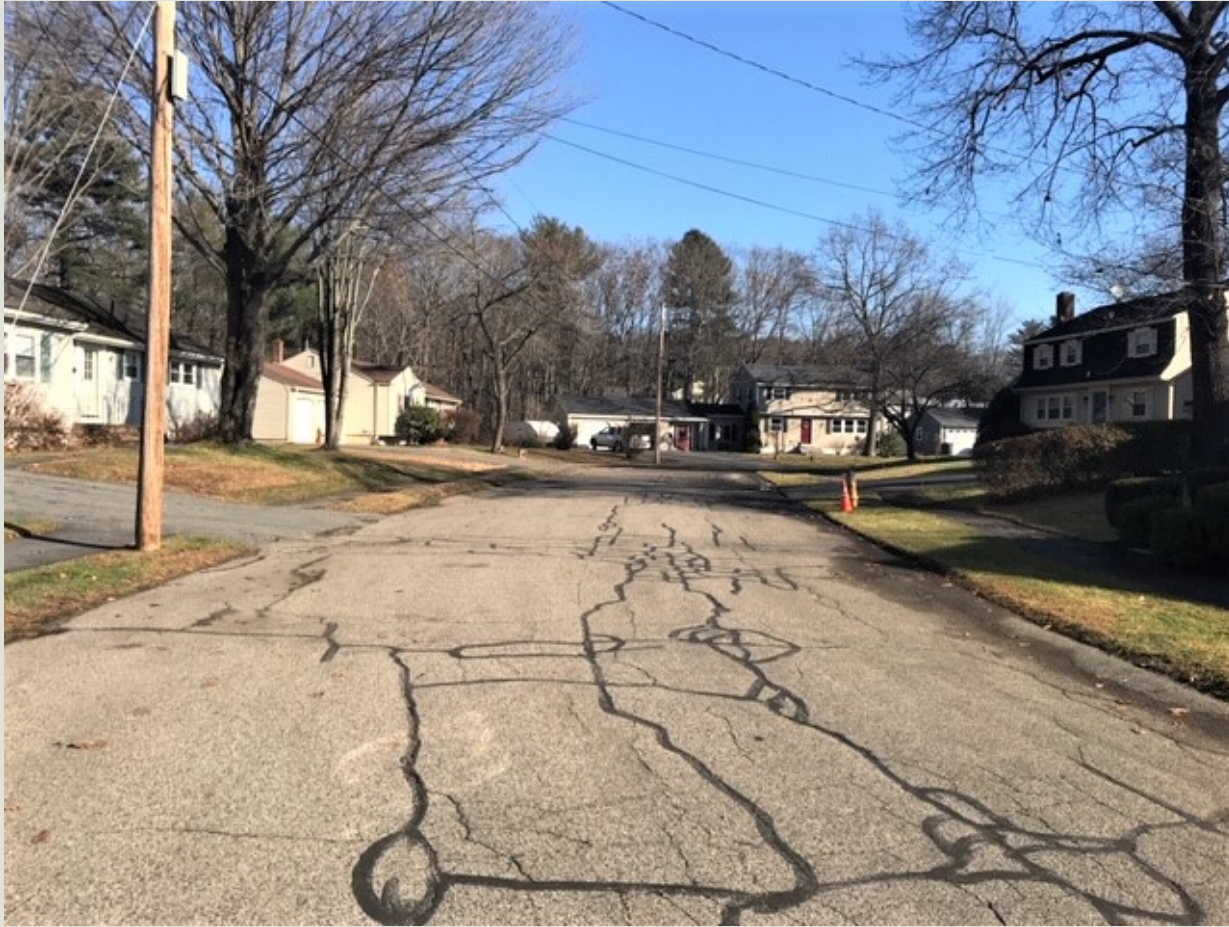
Longwood Drive – PCI = 61; ranked Poor Mill/fill treatment recommendation
