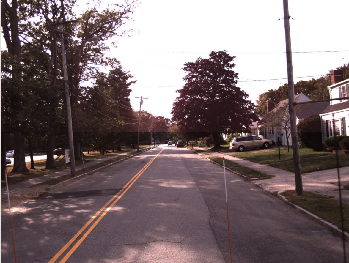
Walton Street – PCI = 83; ranked Fair 1.5" overlay treatment recommendation
