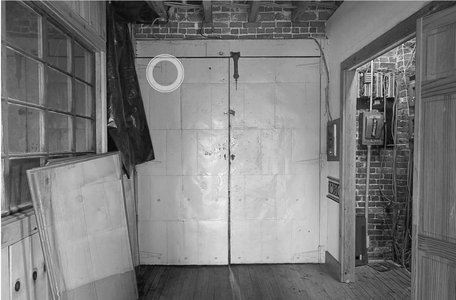
BLDG 6A: STEEL DOORS THIRD FLOOR
