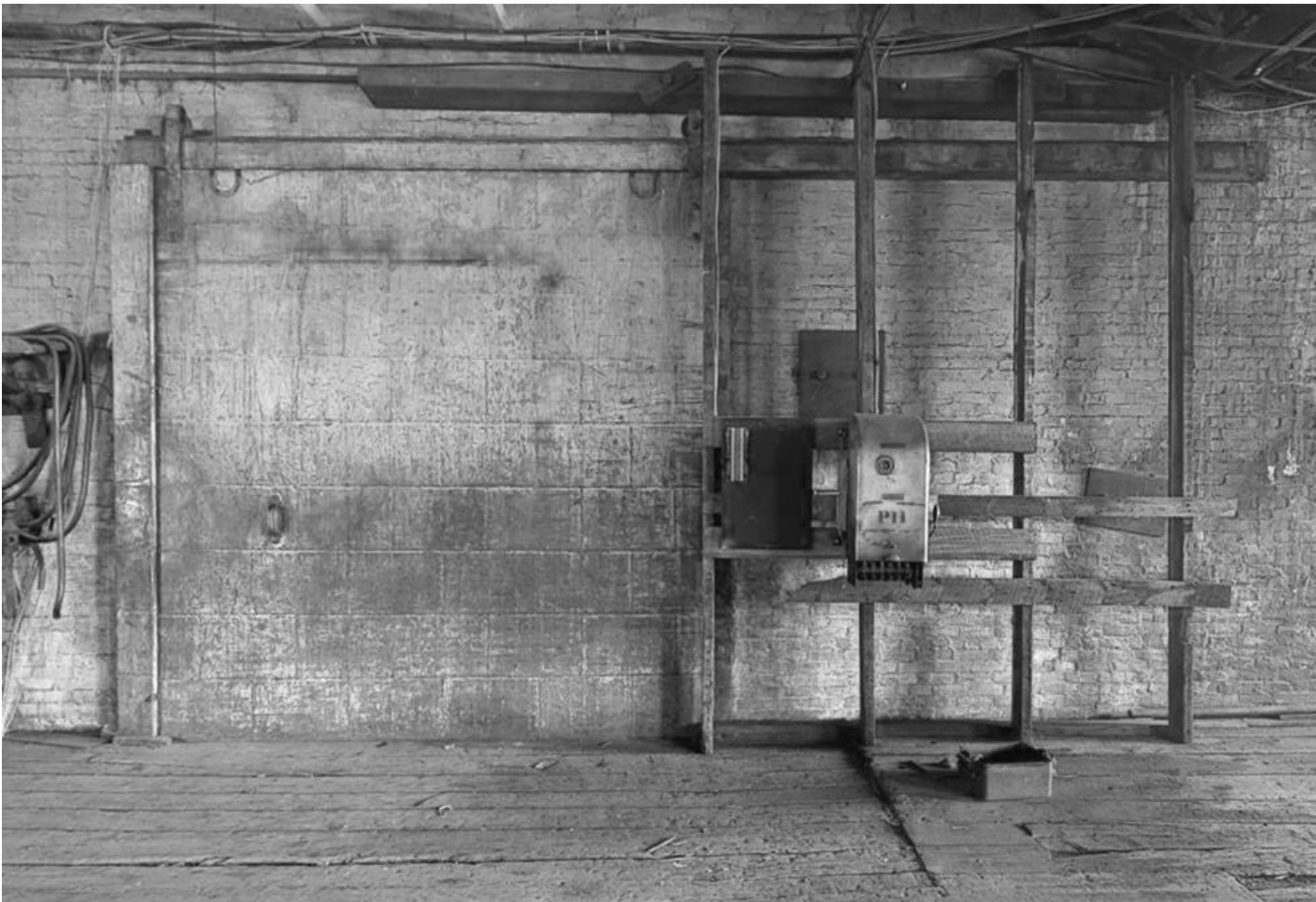
BLDG 3: STEEL SLIDING DOOR, SECOND FLOOR, EAST ELEVATION
