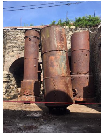
Tank, boilers, vaults and seawall in Building 15
