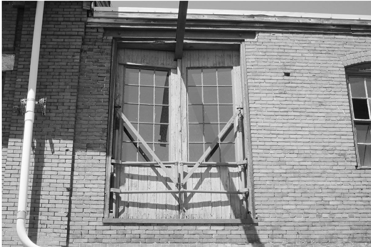
BLDG 2: REBUILD WOOD DOORS & SALVAGE METAL BRACES SOUTH ELEVATION, SECOND FLOOR
