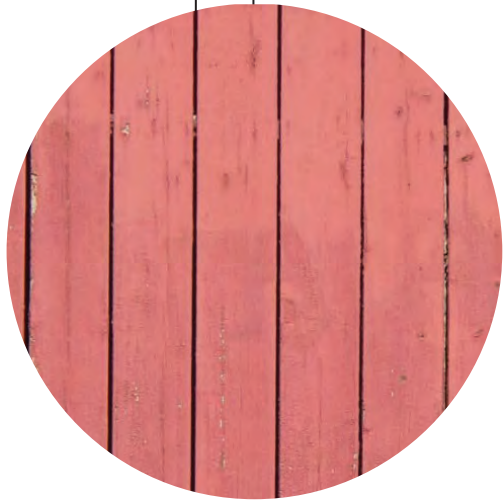
WOOD DOORS & INFILL Painted red wood outer doors and rebuilt wood infill reference previously existing wood infill at oversized openings.
