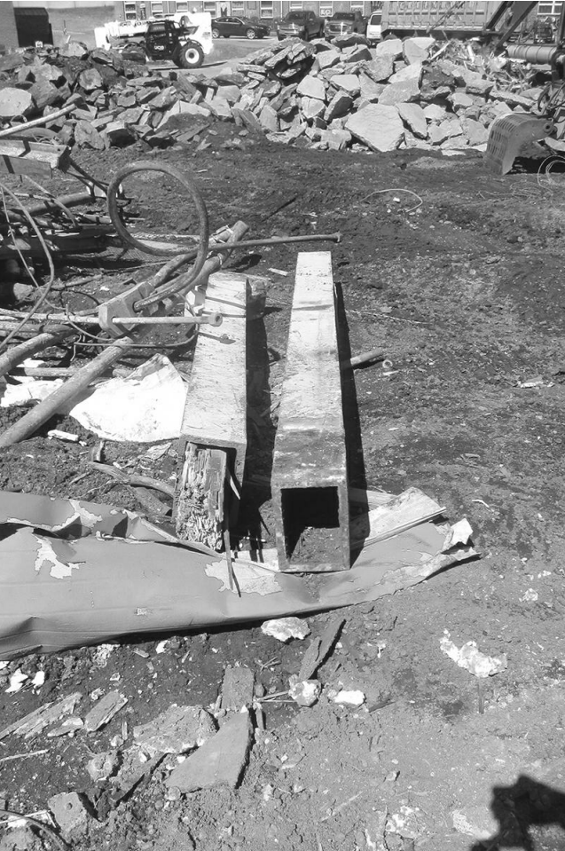
BLDG 6A (FROM BLDG 7): CAST IRON COLUMNS FOR USE AT ENTRY CANOPY
