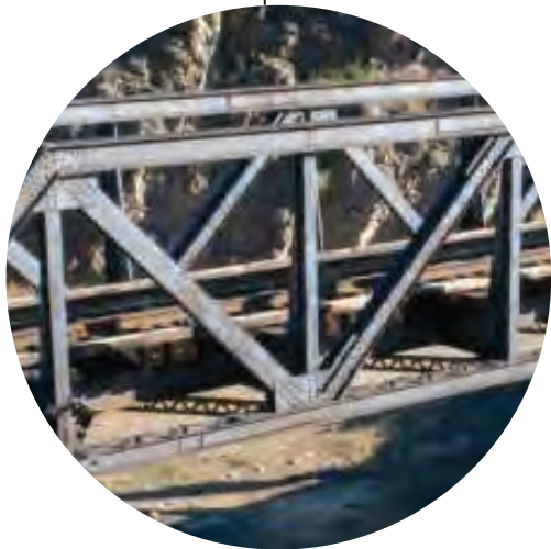
RAILROAD TRUSS Painted railroad truss bridges with corrugated metal roofs and internal picket railings.
