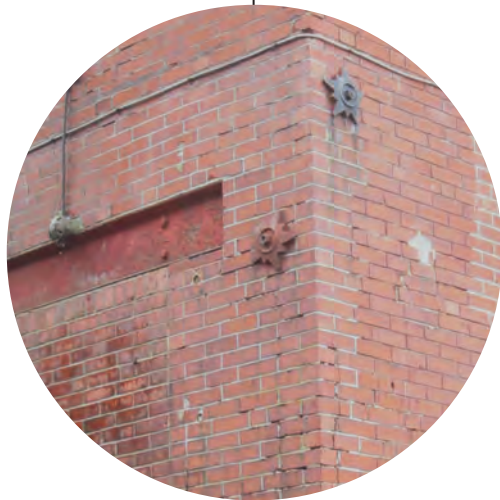
RESTORED BRICK Masonry remaining at Building 2/3 will be repaired.
