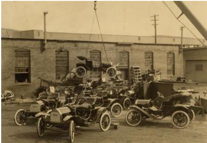
Crane hoist and cars at entrance yard
