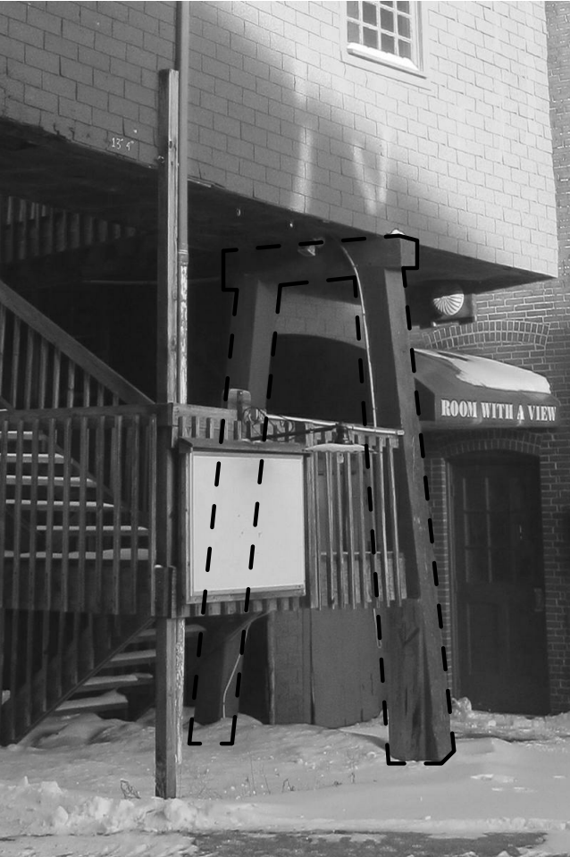
BLDG 6 BRIDGE: WOOD BRIDGE SUPPORT
