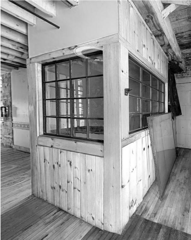
BLDG 6A: ELEVATOR MACHINERY THIRD FLOOR
