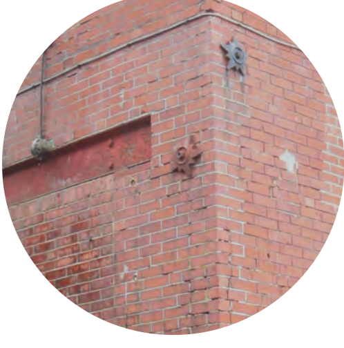
RESTORED BRICK Masonry remaining at Building 24, Building 15, and Building 16 will be repaired.
