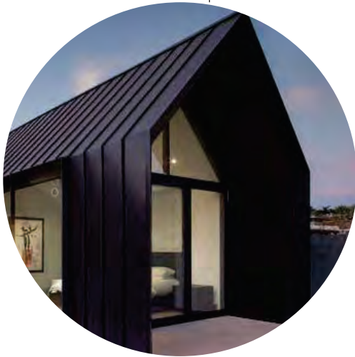
METAL SIDING AND ROOF AT SECONDARY ENTRANCE.
