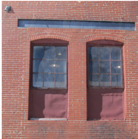
Building 6 - Existing Openings
