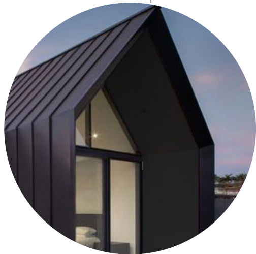
METAL SIDING AND ROOF AT SECONDARY ENTRANCE.
