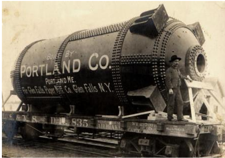
Sulfite digester assembled in Building 6
