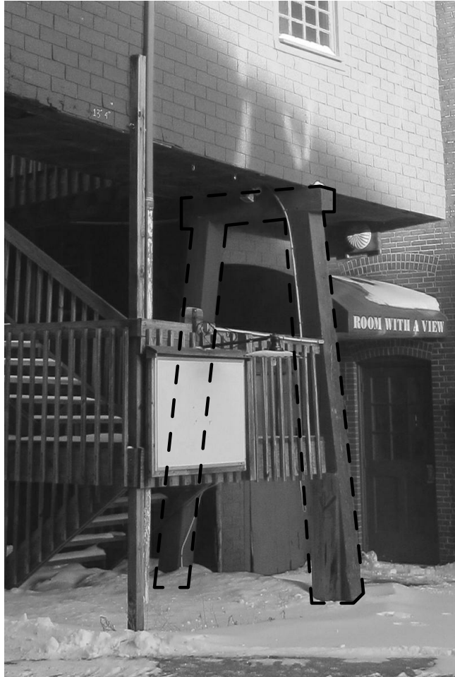
BLDG 6 BRIDGE: WOOD BRIDGE SUPPORT
