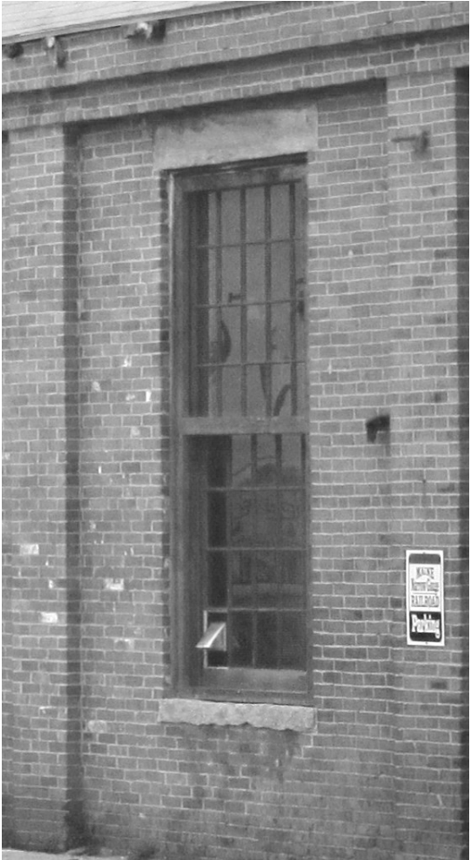
BLDG 6B: WITNESS WINDOW
