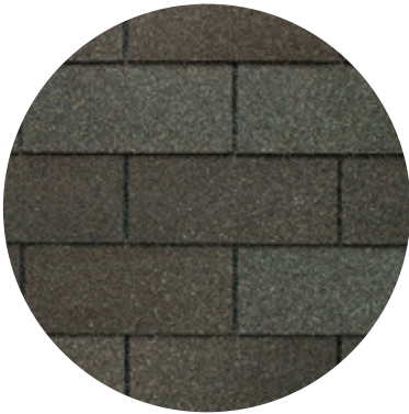
THREE-TAB ASPHALT SHINGLE AT PITCHED ROOF
