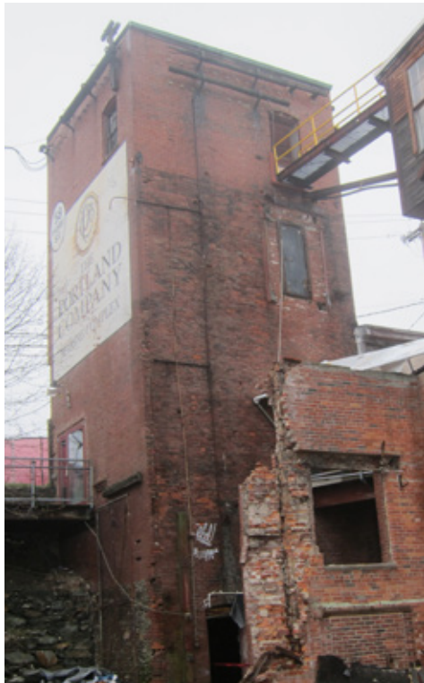
Building 24 - Existing Conditions
