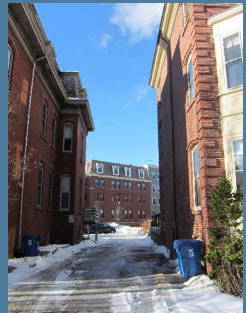
Rear as viewed from Pine Street
