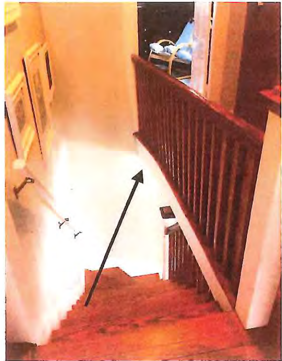
UNUSUAL. STEAM BENT BOARD, SHAPED TO THE SPACE. FEELS LIKE BEING ON A SHIP. JAMES B NEWELL WAS A JOINER WHO BUILT THE HOUSE,
