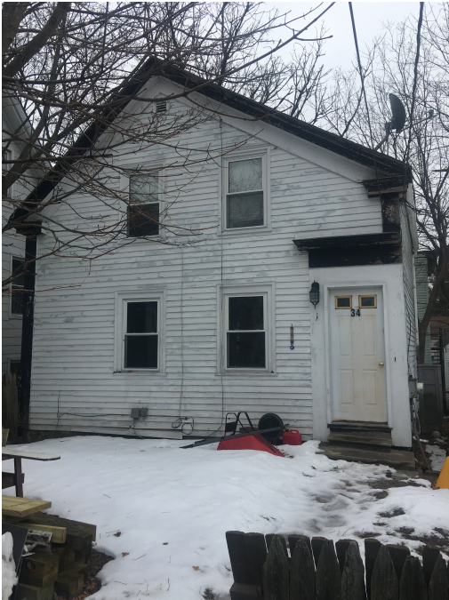
Photo #1 view of exterior of building
