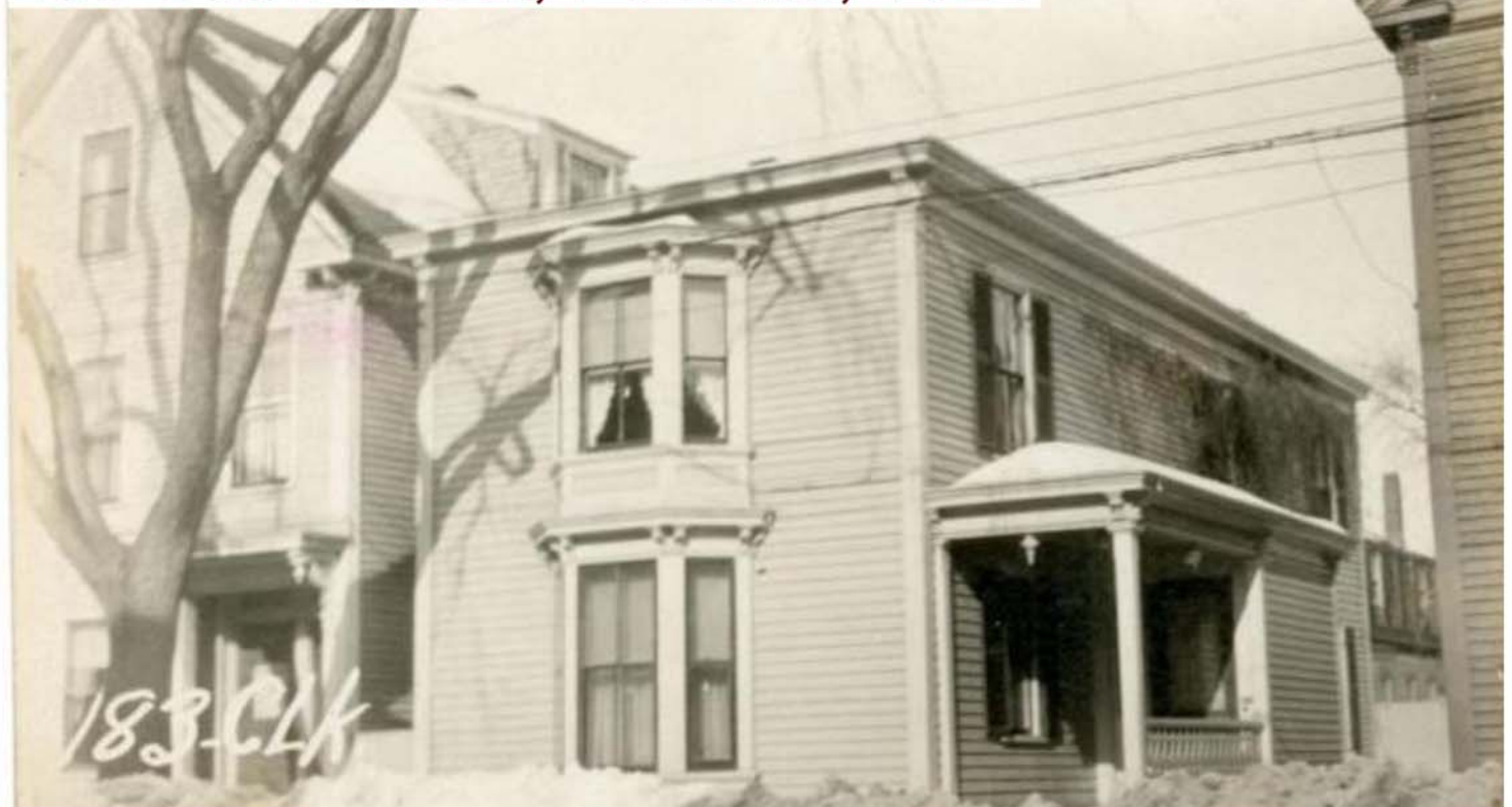
183 Clark Street, Portland, 1924
