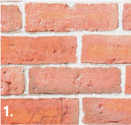
1. LOCATION: All exterior walls with exception of north elevation infill.
