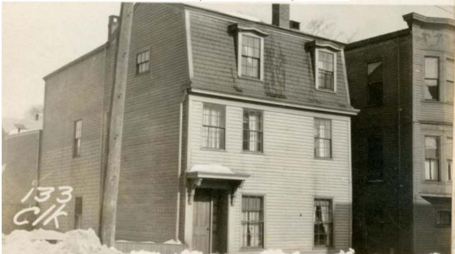
131-135 Clark Street, Portland, 1924
