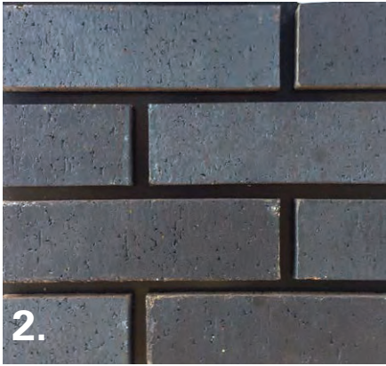
2. LOCATION: North elevation infill.
