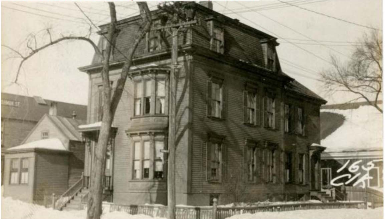
165 Clark Street, Portland, 1924
