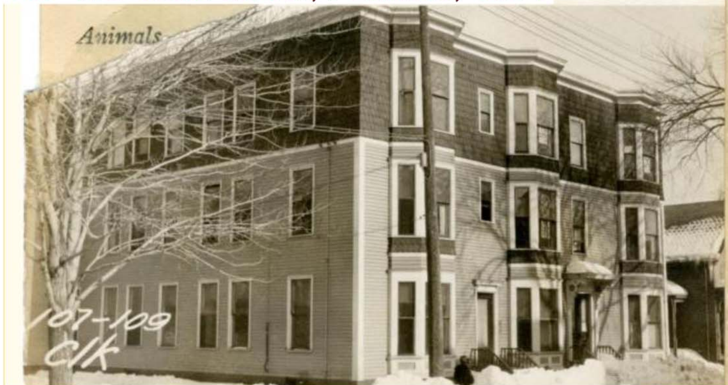
107-113 Clark Street, Portland, 1924
