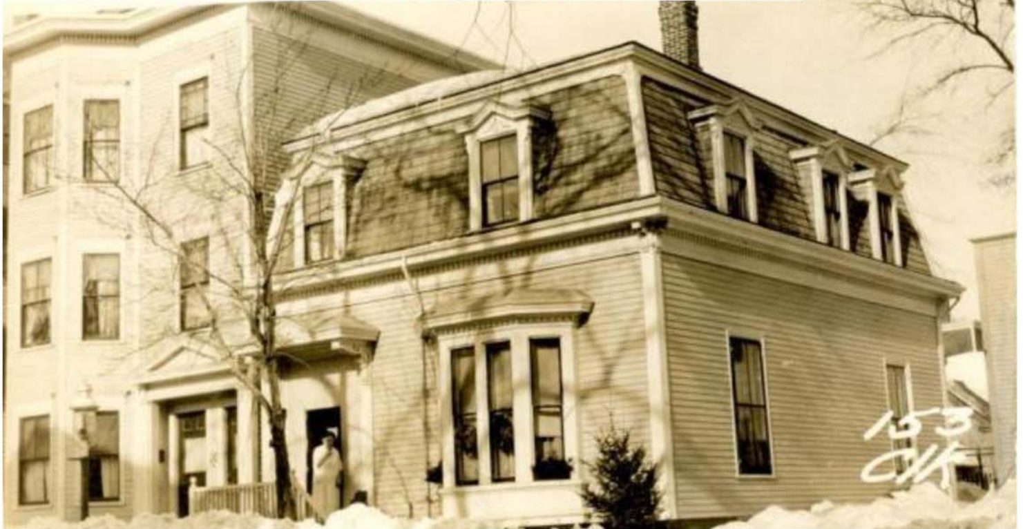
151-155 Clark Street, Portland, 1924
