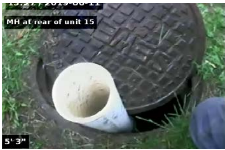
entrance to sewer mahole 1
