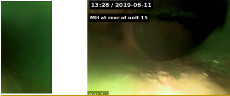
Line view at sewer wye
