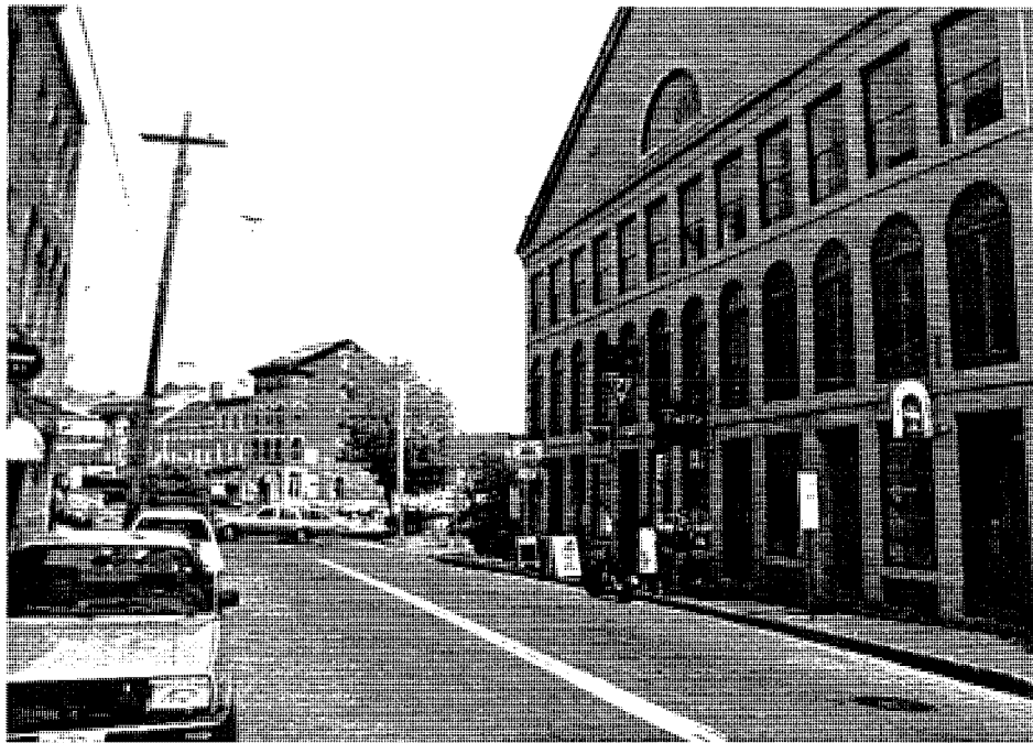
South side of Fore Street.
