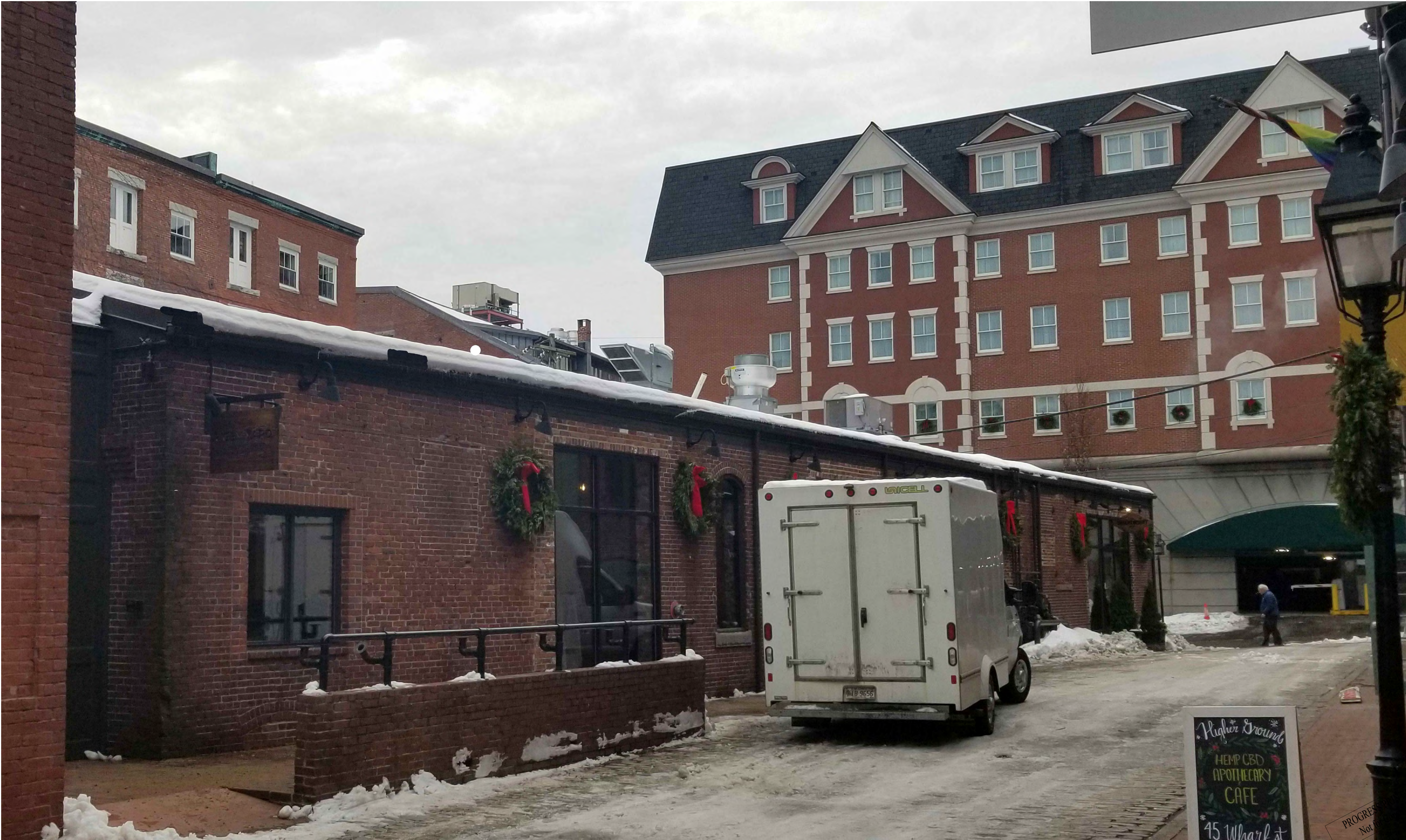
1 VIEW LOOKING SOUTH ON WHARF STREET (BEFORE) N.T.S.
