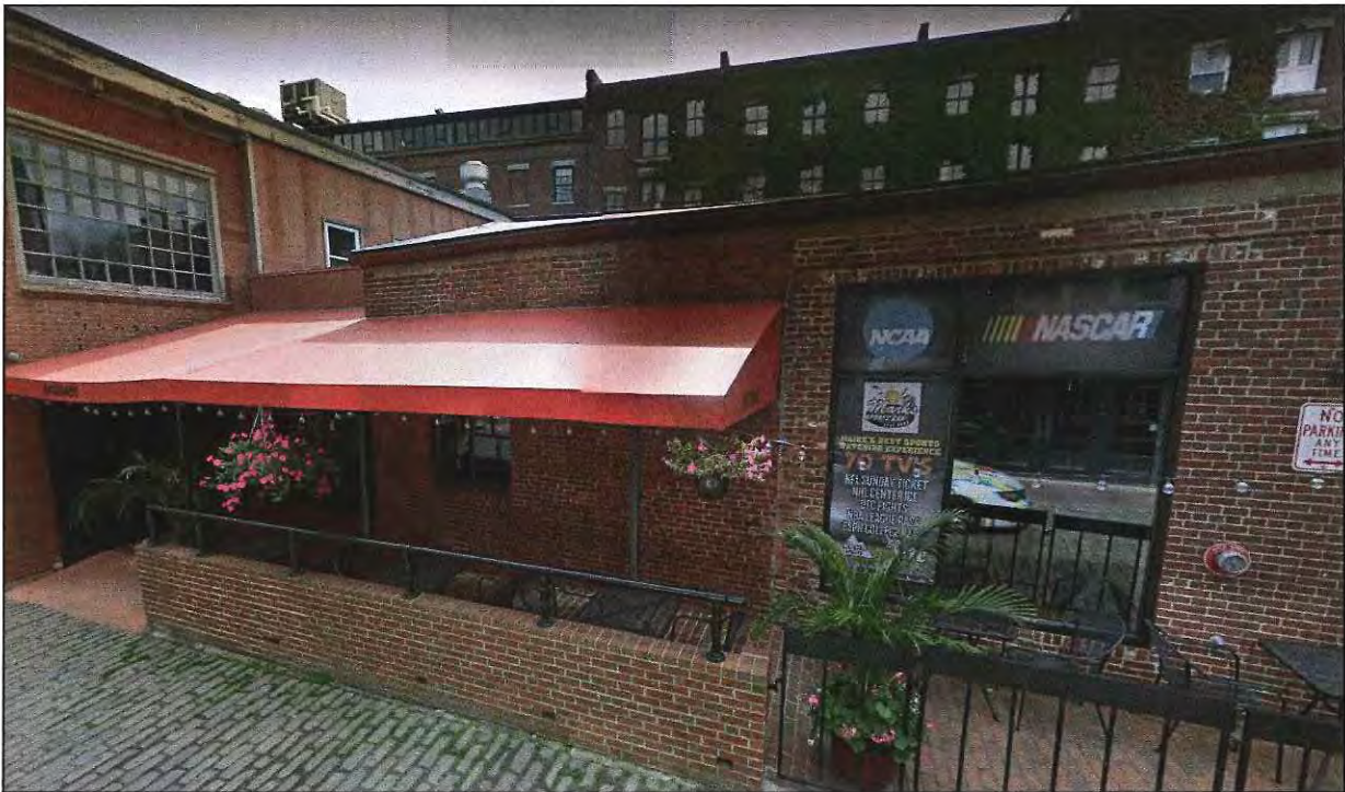
4 EXISTING VIEW LOOKING EAST ON WHARF STREET
