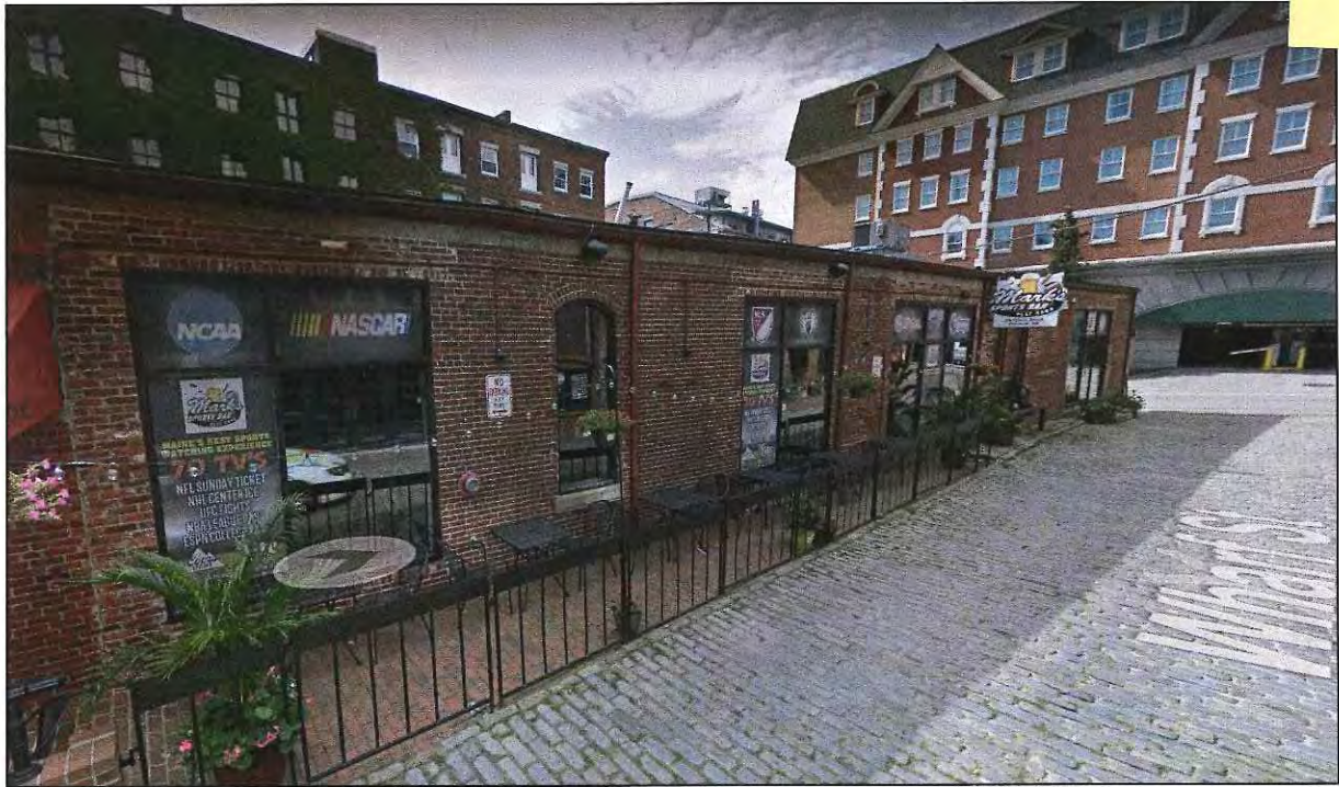
2 EXISTING VIEW LOOKING WEST ON WHARF STREET
