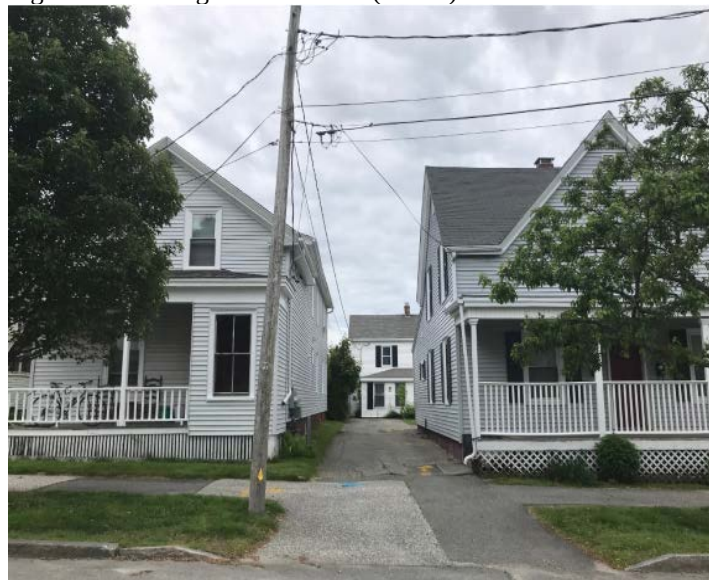
Figure 2 - Existing 126 and 128R (at rear) North Street
