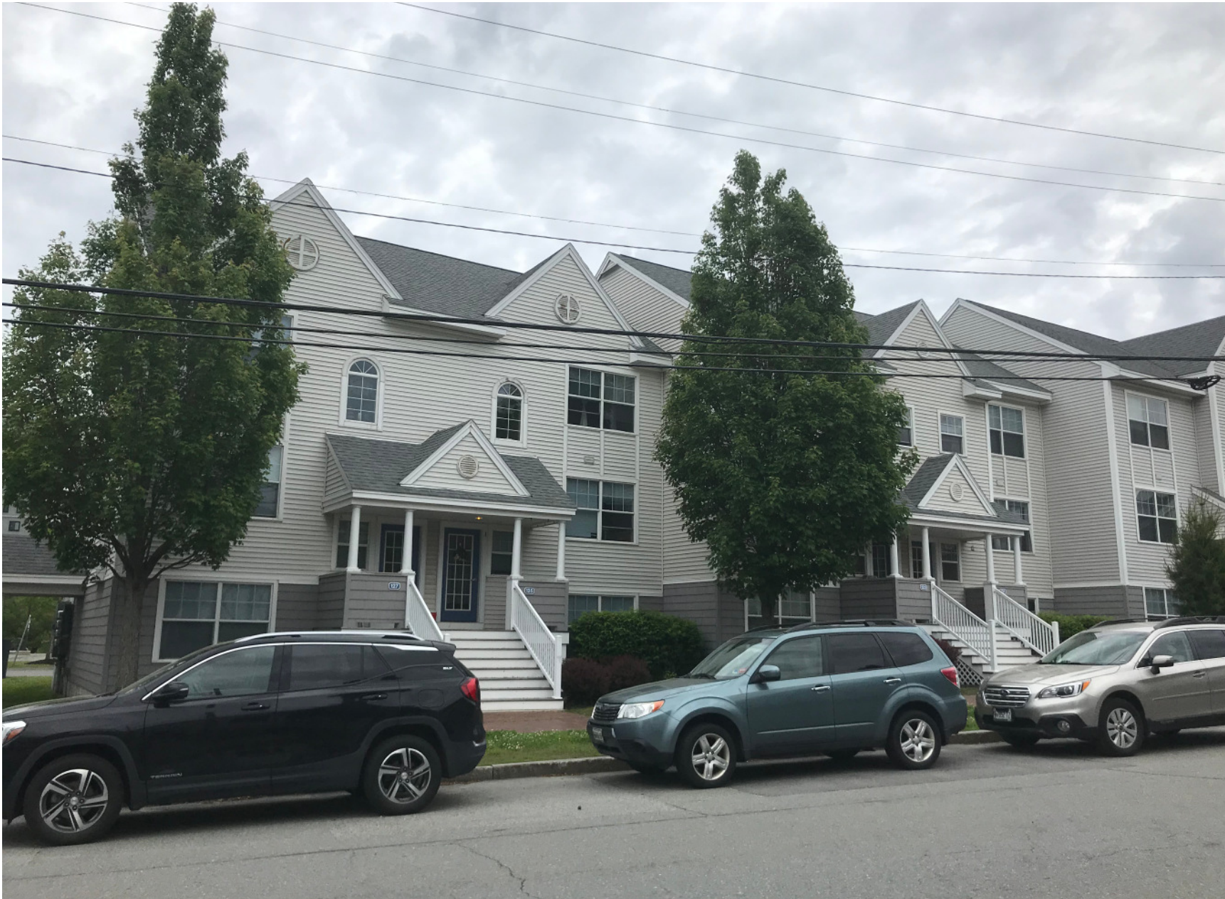
A section of Island View Apartments across the street. The complex has a mixture of single and mulled windows and is clad in clapboard-style lap siding. Parts of the complex are three stories high and some sections are four stories.
