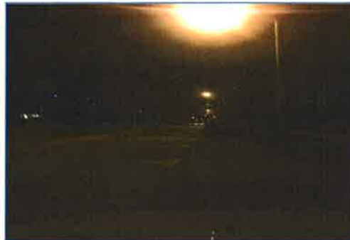
Baltimore Before – HPS Cobra Head Luminaires
