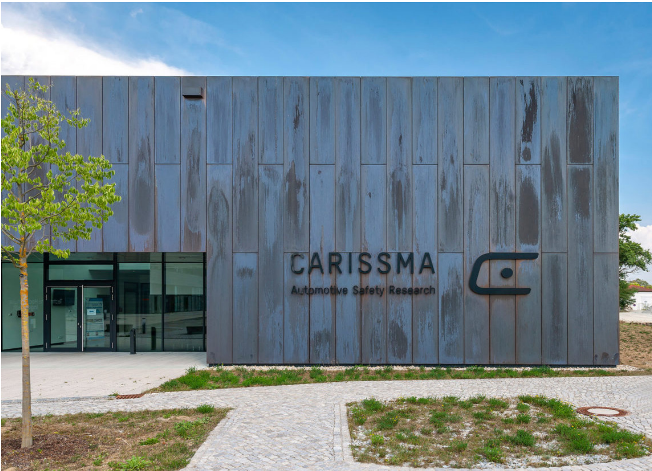
CLADDING TYPE 2: COPPER PANEL 'GRAPESKIN' LIVE FINISH
