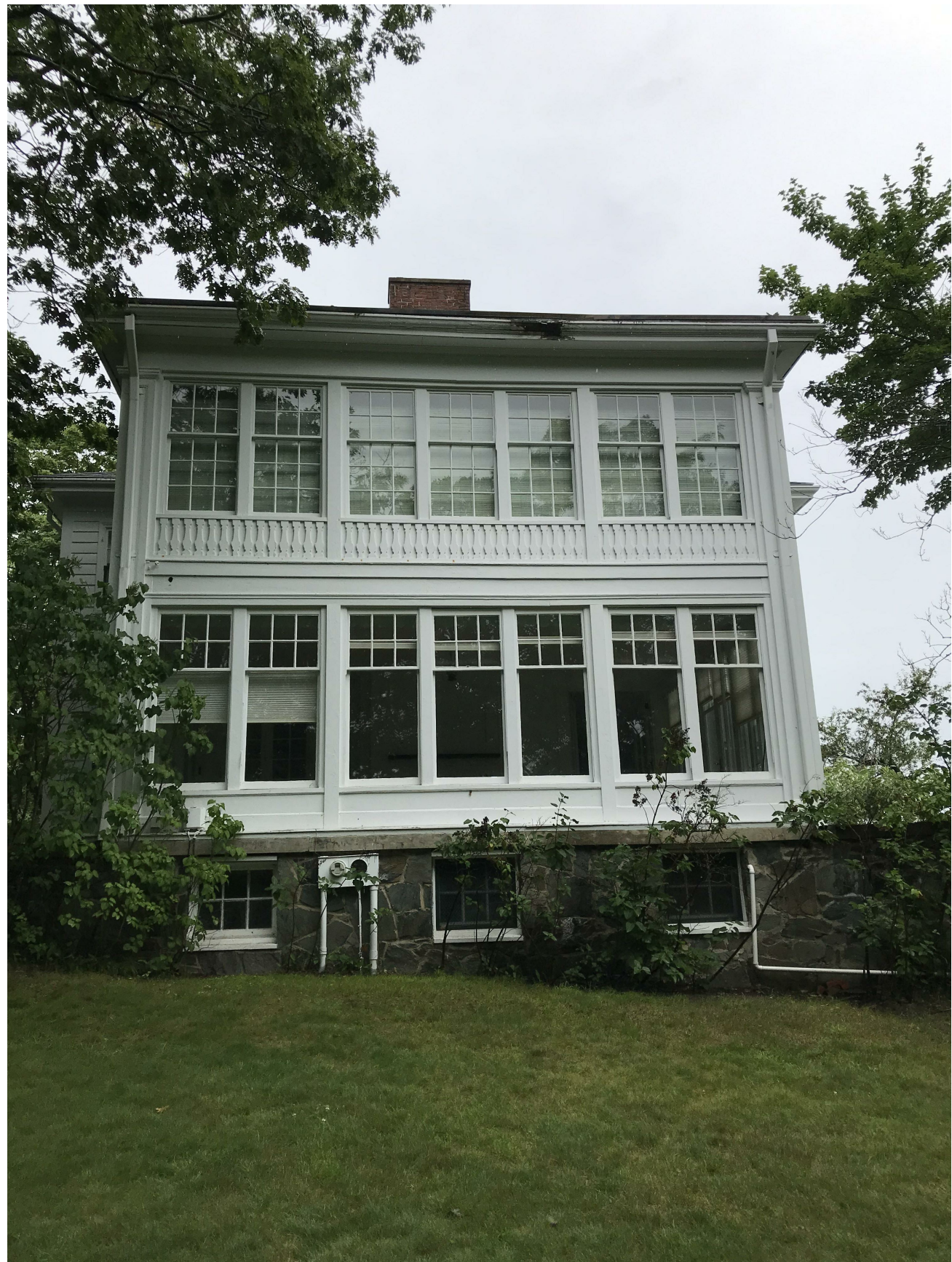
TWO STORY SUN PORCH AND THIRD FLOOR ROOF BALUSTRADE
