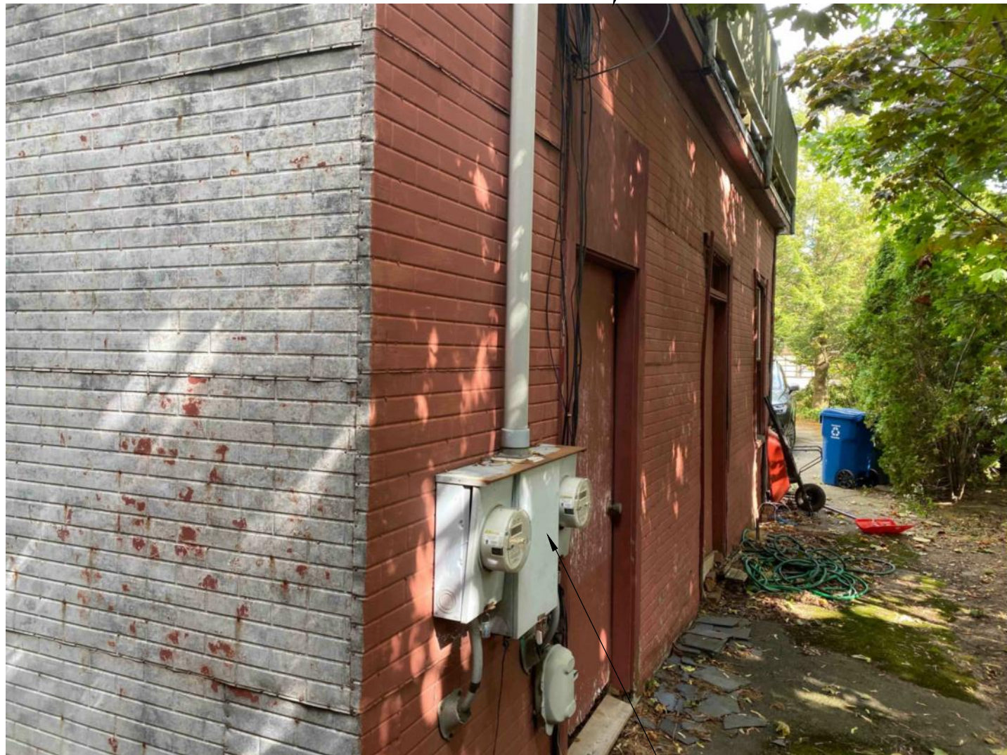
11 NOTHERN VIEW OF GARAGE
