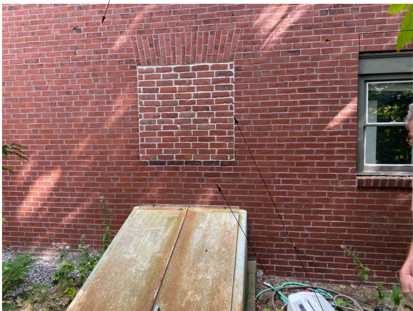
8 WESTERN BULK HEAD VIEW
