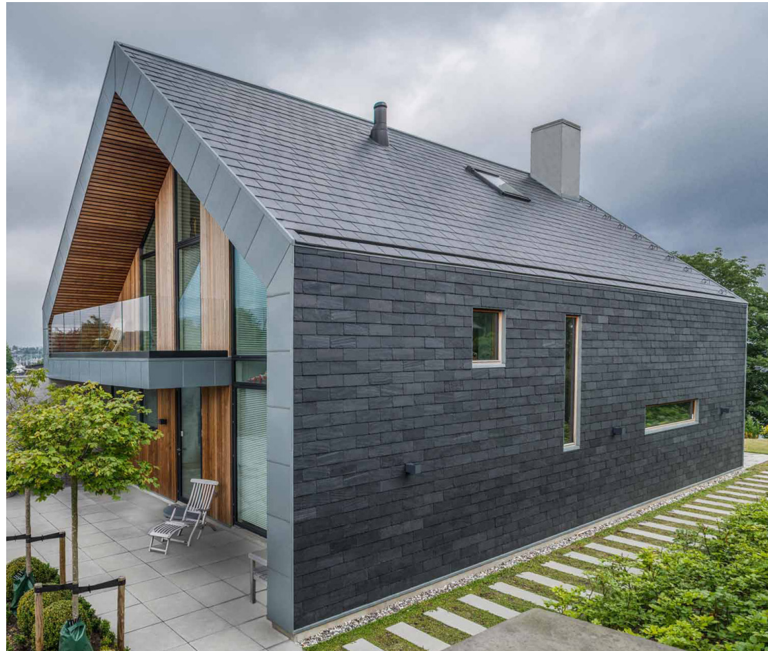
CLADDING TYPE 1: SLATE SHINGLE (NOTE INTEGRAL GUTTER)
