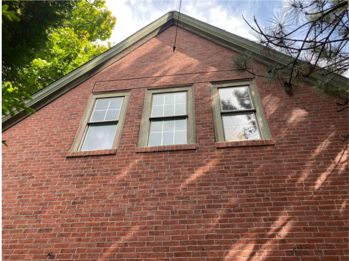
9 WESTERN VIEW OF GABLE
