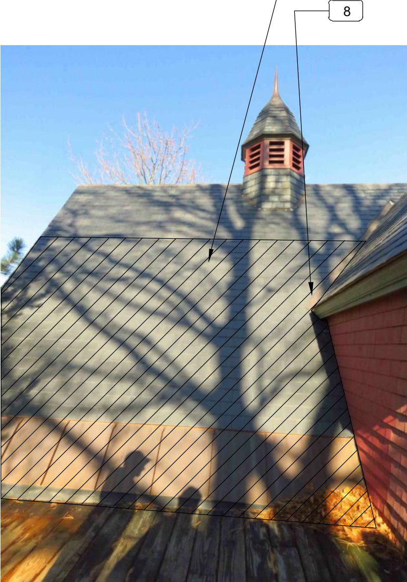
4 VIEW OF ROOF TO BE REMOVED
