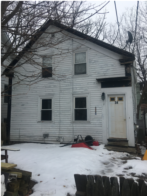
Photo #1 view of exterior of building
