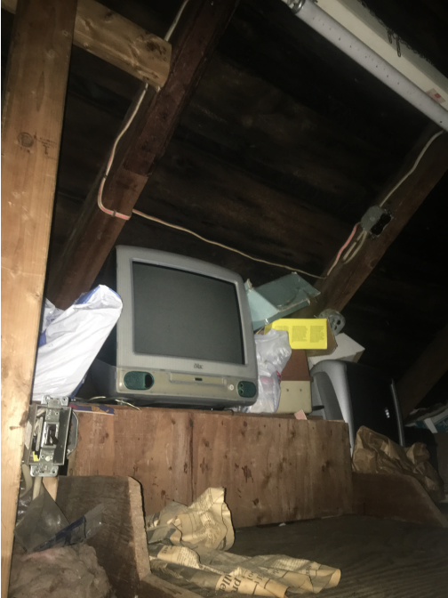
Photo #4 of Attic space
