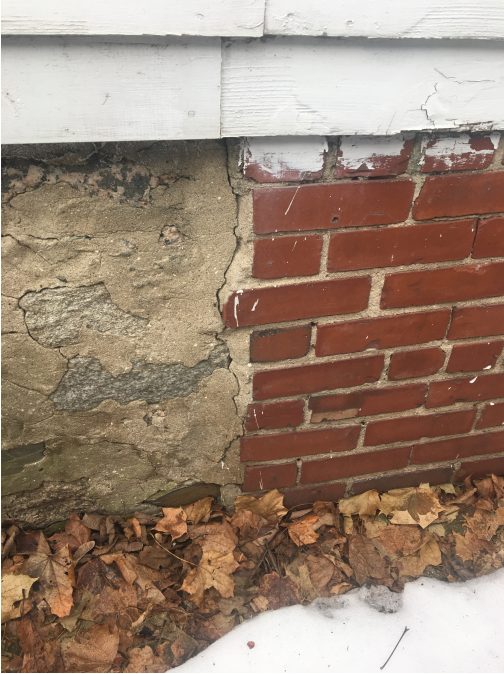
Photo #2 close up view of exterior showing foundation
