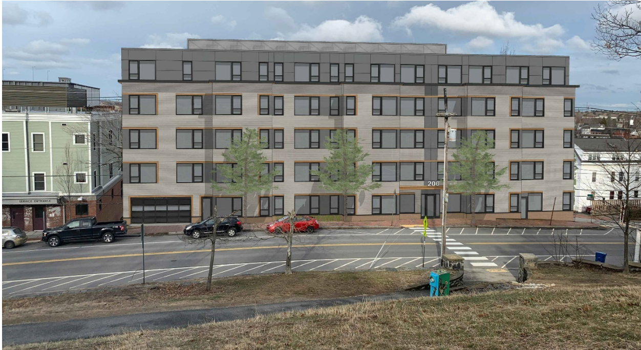
Figure 3: View Looking from Walking Path - Source: Ryan Senatore Architecture
