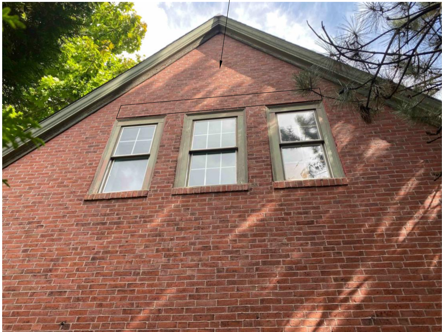
9 WESTERN VIEW OF GABLE
