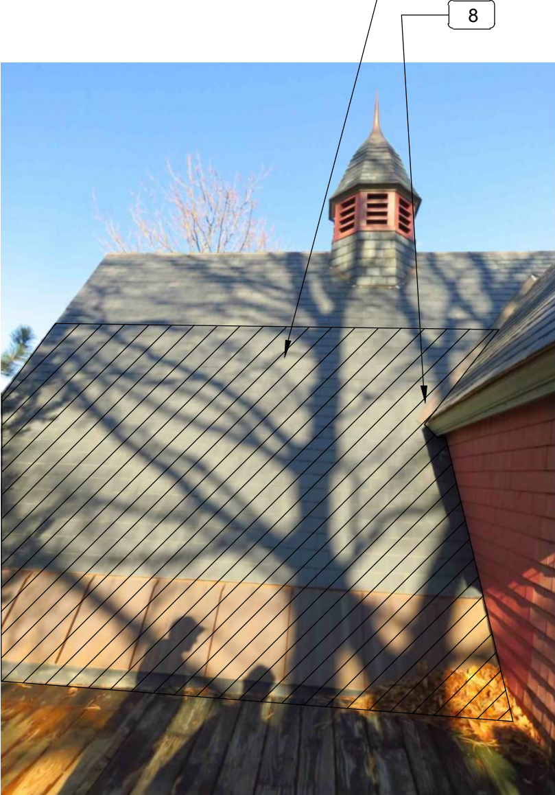
4 VIEW OF ROOF TO BE REMOVED
