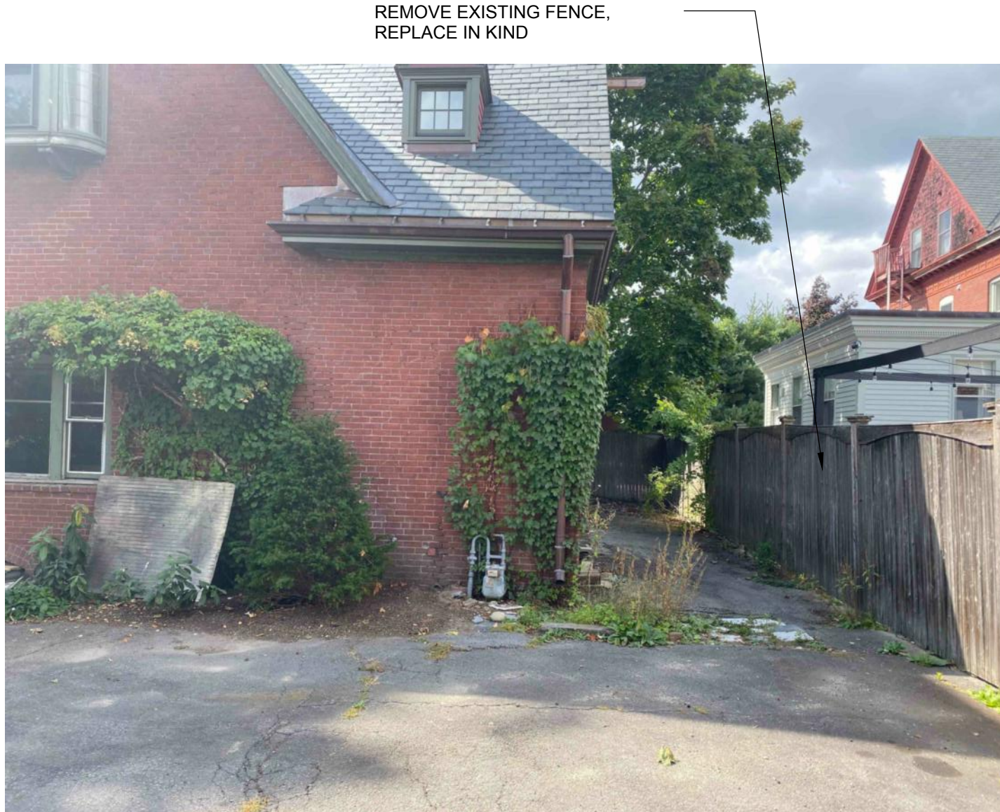
7 VIEW OF EXISTING FENCE
