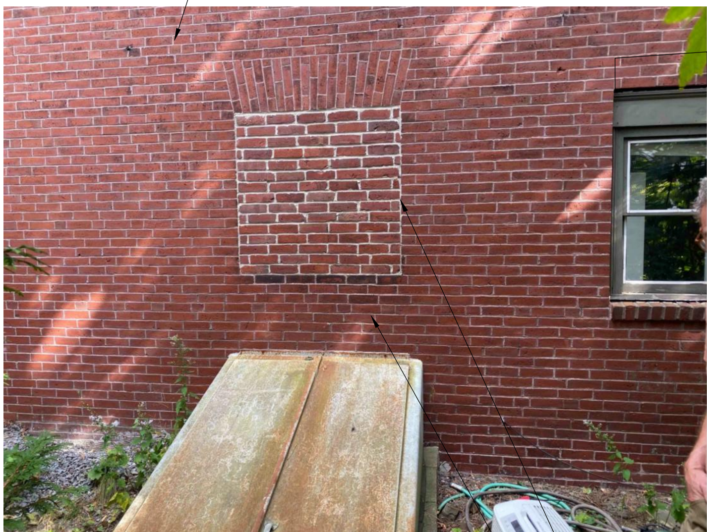
8 WESTERN BULK HEAD VIEW
