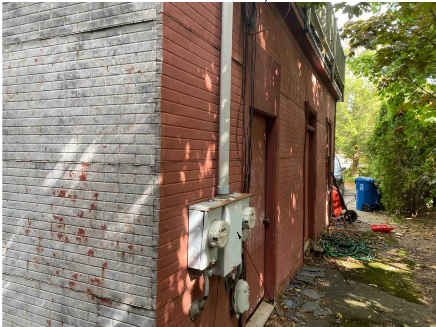
11 NOTHERN VIEW OF GARAGE
