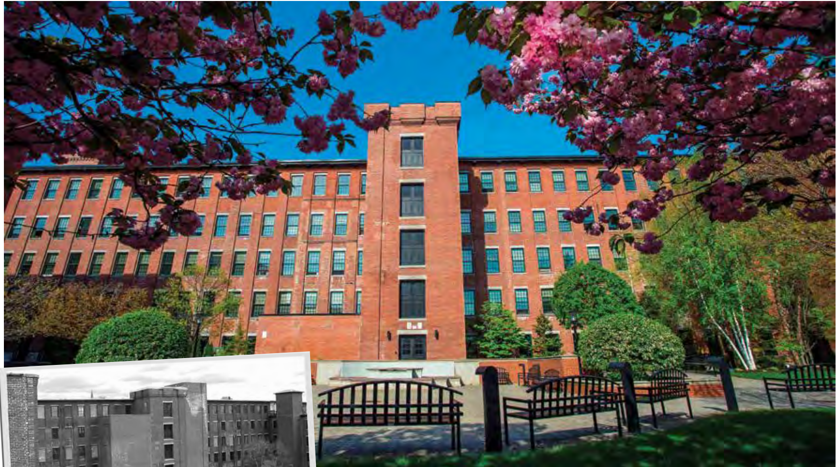
Bottom Left: The Lofts at Bates Mill, west facade and Fountain Park, before Above: Same view, after renovations
