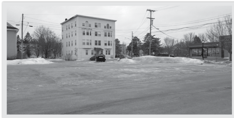
Above: Rendering of completed project Left: Same location, prior to construction
