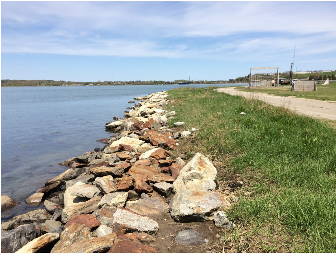
Photograph 1. View looking northeasterly at rip rap bank and Back Cove. 05/16/18.
