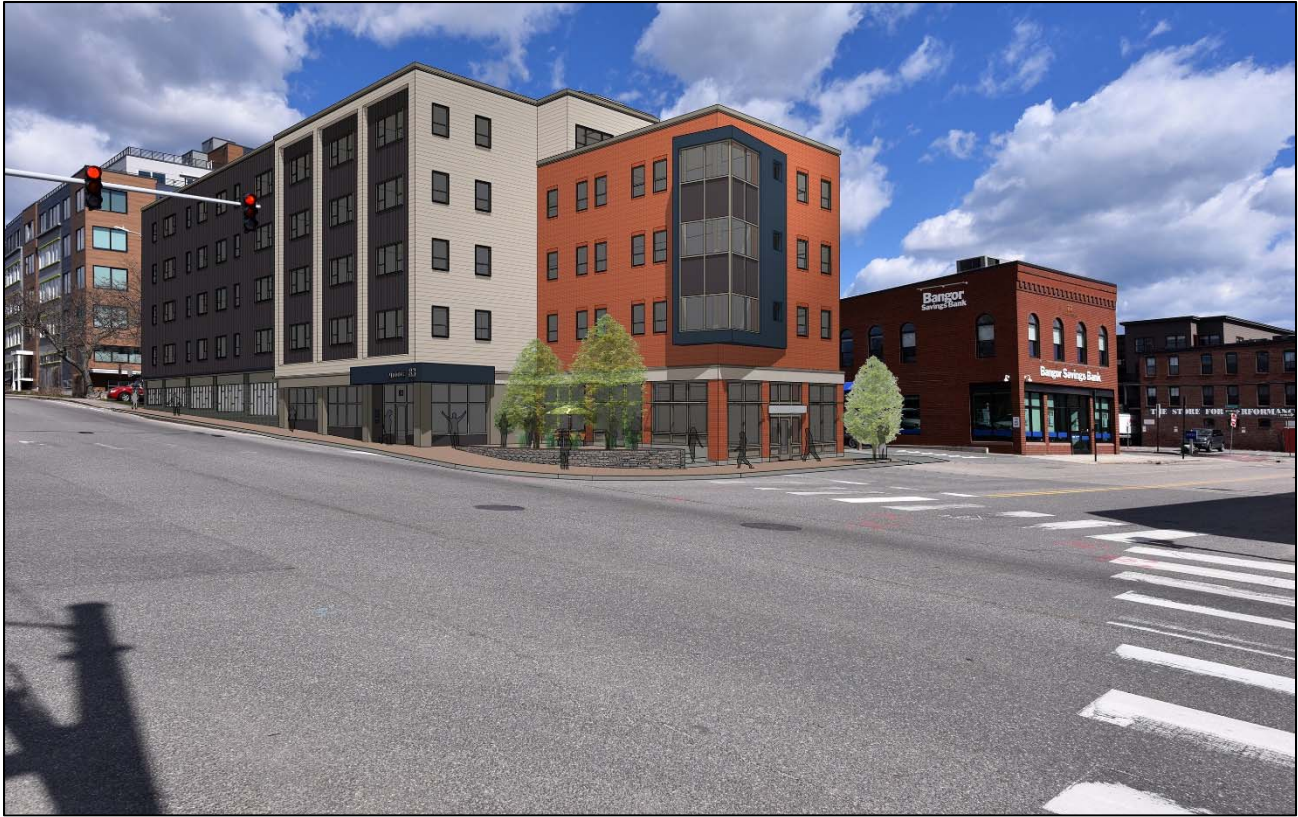
Figure 3 View of Project from Franklin St
