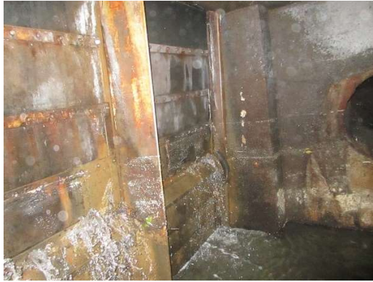
Looking downstream tide gate and 30" SD Inlet
