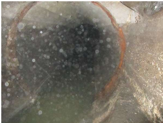
Looking upstream at 96" RC Inlet
