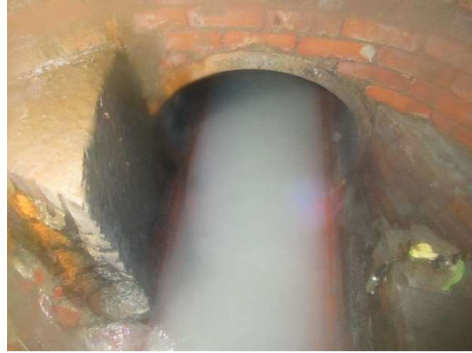
View looking upstream at 30" VCP inlet
