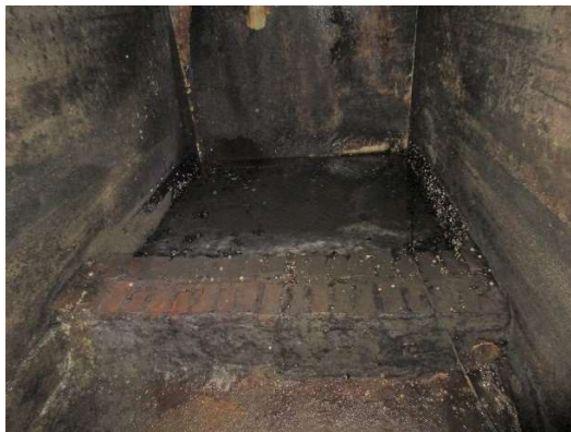
View looking downstream toward tide gate
