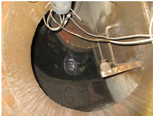
View looking down into concrete chamber
