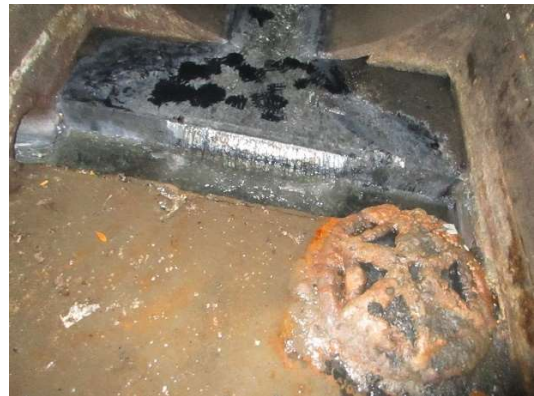
View looking upstream at 72" RC inlet
