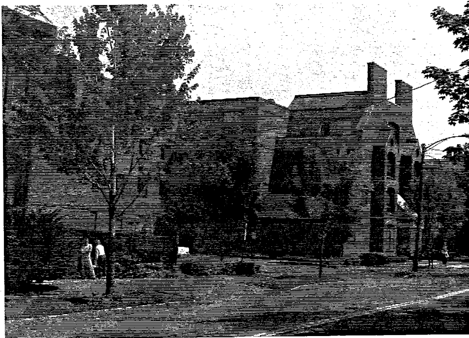
The four story height of this Cumberland Park Place apartment complex is reduced at the sides and front of the building by pitched roofs, projecting banks of windows, and other details that attract the eye to lower parts of the building. The composition of the facade can be broken into subgroupings, some of which are of the same scale as the adjacent houses.
