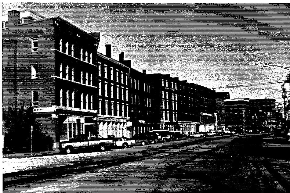
North side of Commercial Street.
