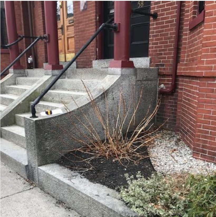
Residence at 56 Thomas Street with 12" W x 12" Ht. granite curbing as a wall.
