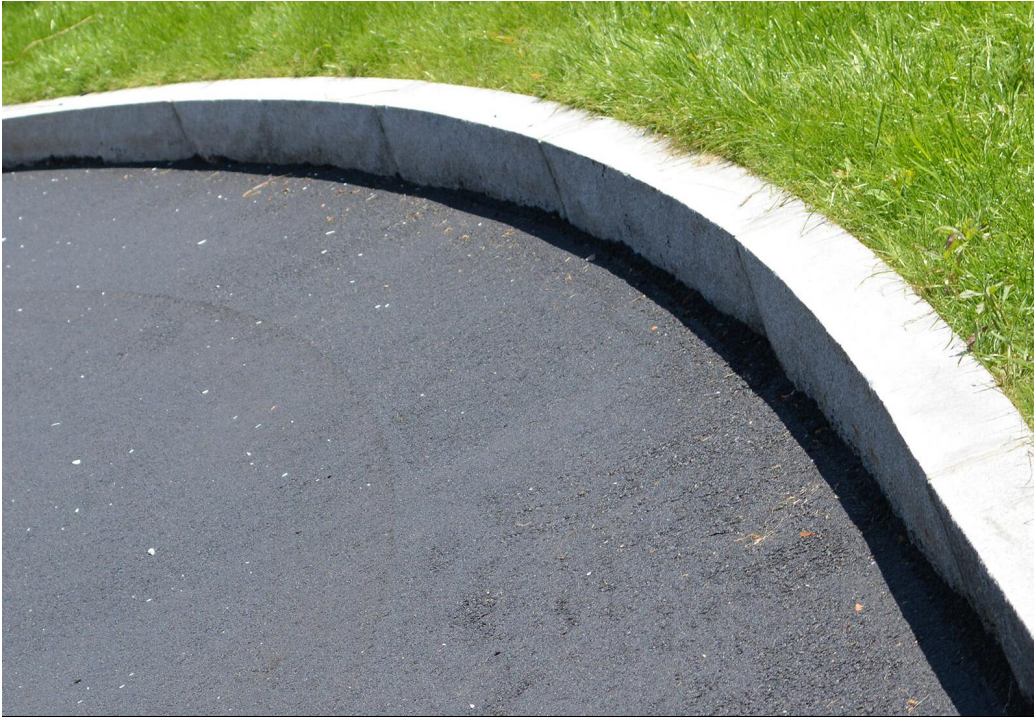
10" Wide Granite Curbing To Replace Timber Wall
