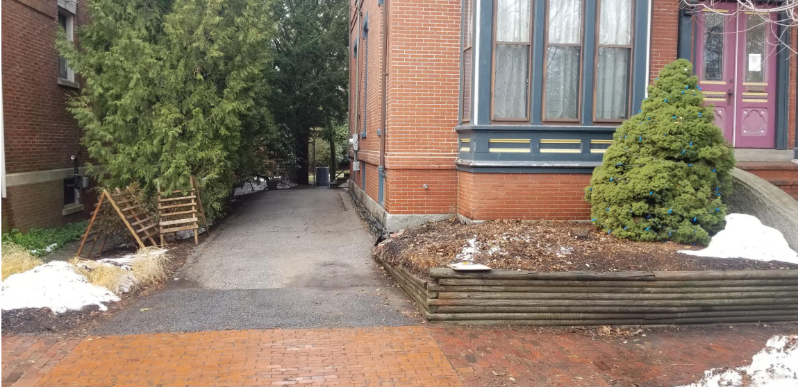
Existing view of driveway and bordering wooden timber retaining wall.
