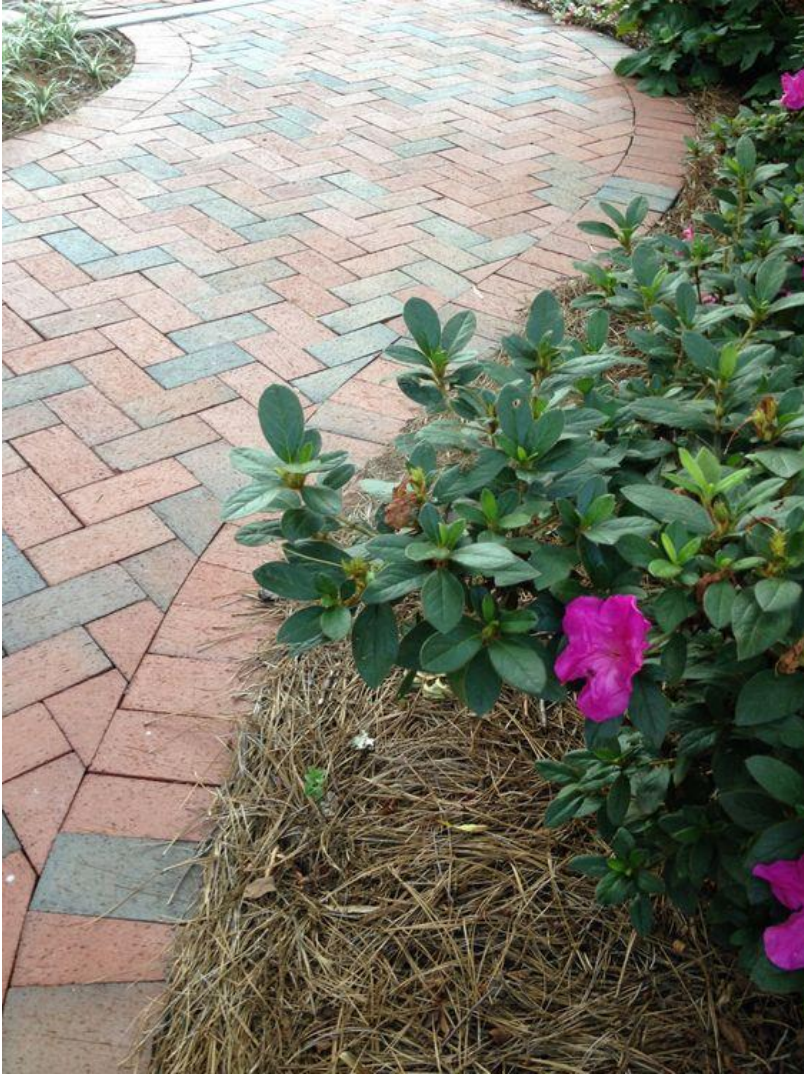
Pinehall Brick Pavers To Replace Asphalt Driveway
