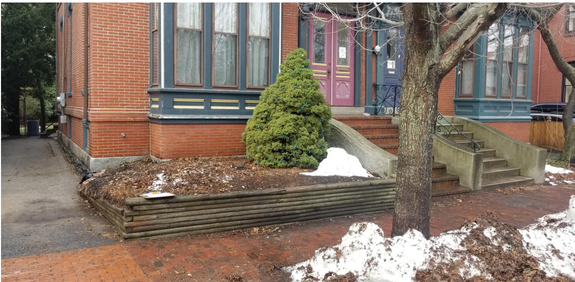
Existing view of front plant bed & wooden timber retaining wall against sidewalk.
