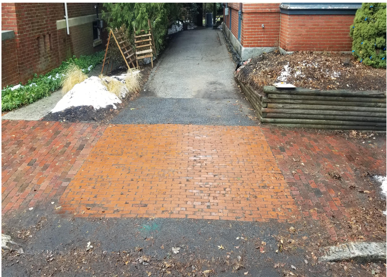
Existing Conditions Of Wall And Driveway
