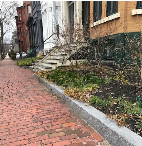
Residence at 1 Carroll St. with a 6" W x 7" High granite curb retaining plant bed.
