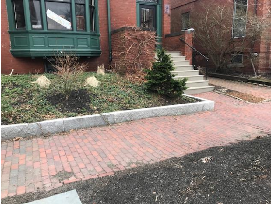
Residence at 19-21 Thomas Street with 6" W x 10" High curbing to retain planting bed.
