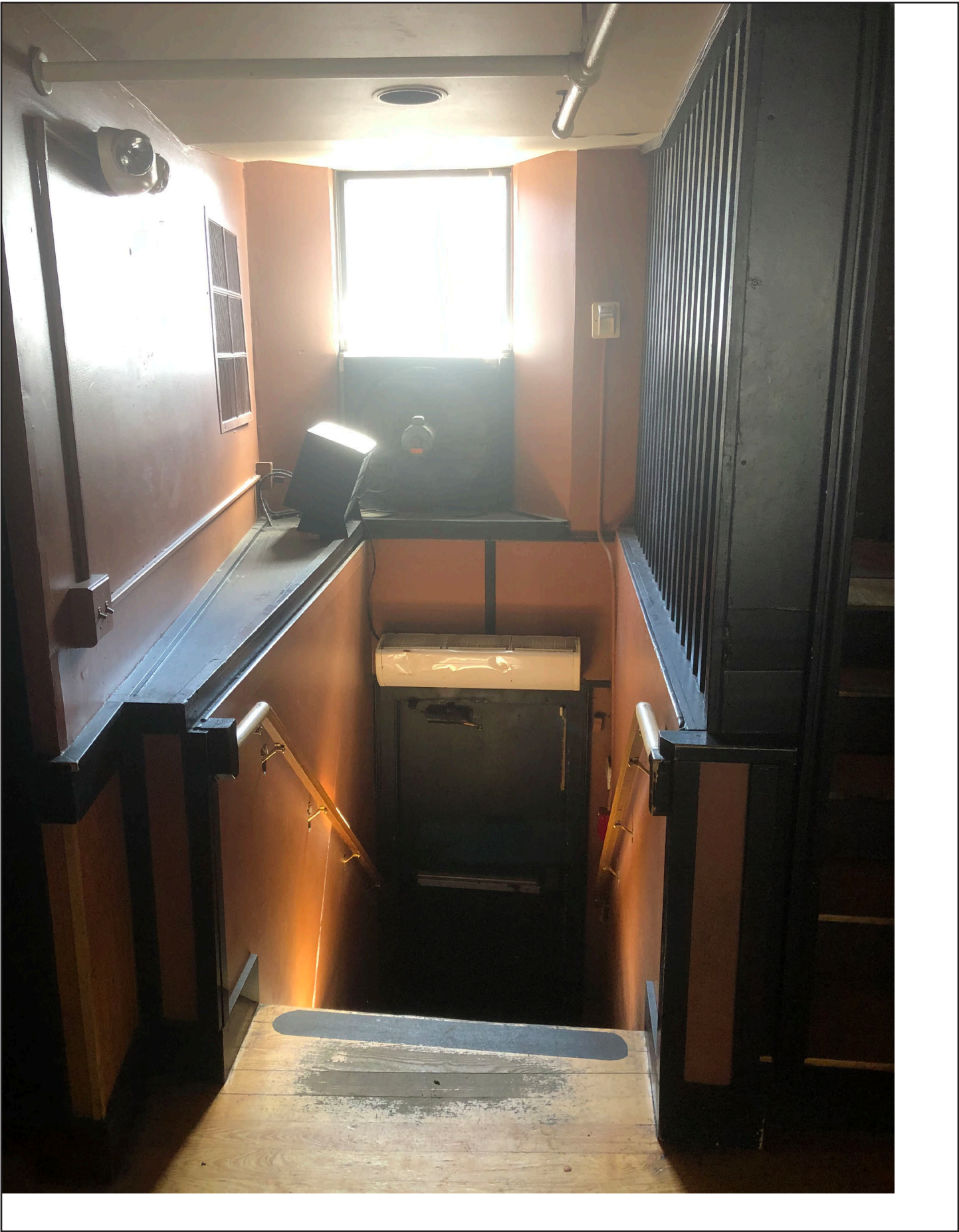
Summer 2020 446 Fore Street Existing door on right from Wharf Street to 1st floor. To be remade into door to basement and ceiling built above
