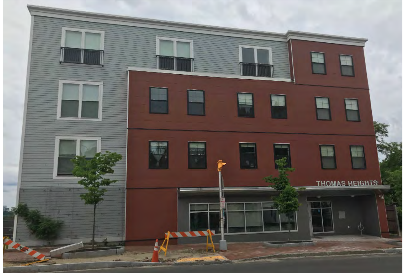
New flat-roofed four-story building along Washington Avenue (at right) and new three story building along Walnut Street.
