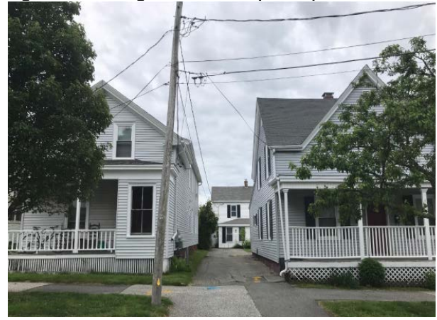
Figure 2 - Existing 126 and 128R (at rear) North Street
