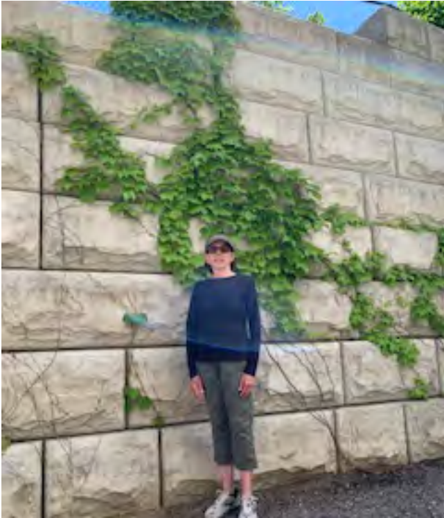
Munjoy Heights Retaining Wall 1
