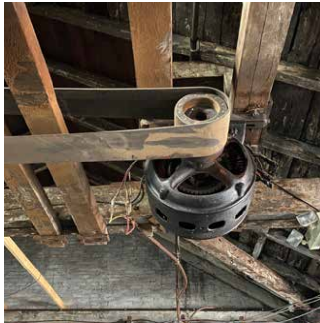
Building 3 / Queen post trusses and machinery
