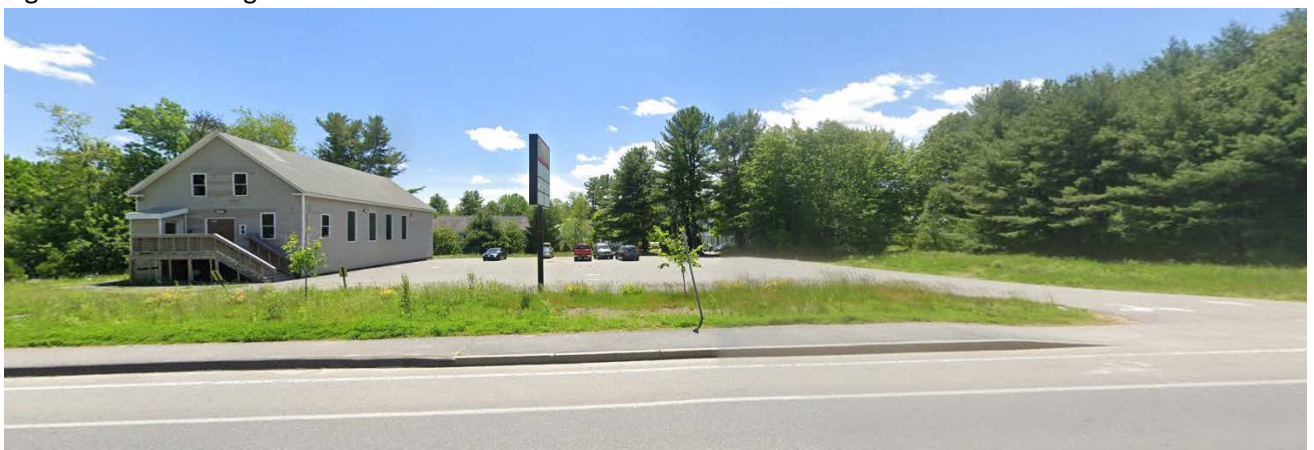
Figure 2: The Existing Site
