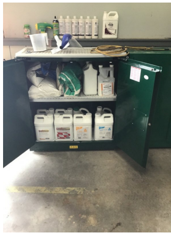
Chemical Storage with Containment
