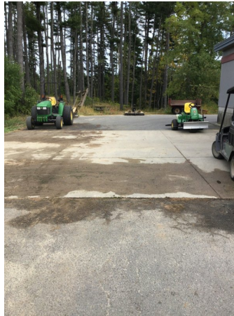
Existing Wash Pad
