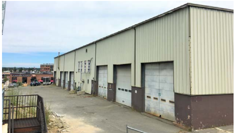
Figure 2: Photo provided by Cushman Transportation Consulting, LLC of West Elevation View along Parris Street view of Existing Building
