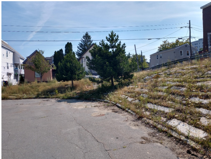
Figure 10. Facing embankment while located along southern edge of site (left portion of embankment pictured is located on site).
