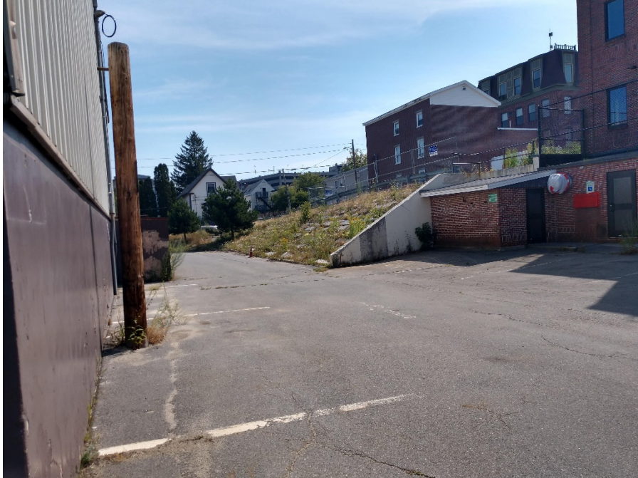
Figure 7. Facing approx. east while located along southern edge of existing building.
