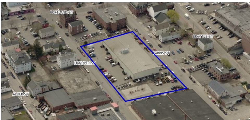
Figure 1: Aerial view (South View) of 52 Hanover Street vicinity with development area highlighted
