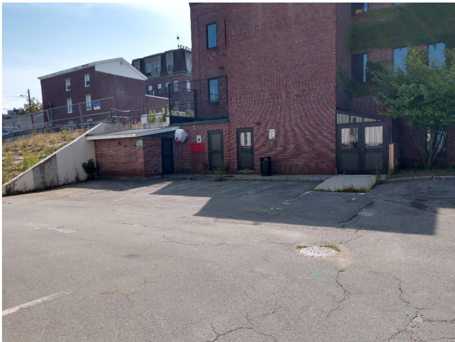
Figure 6. Facing approx. southeast while located near south corner of site.
