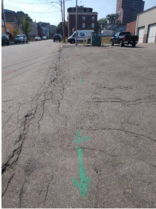
Figure 1. Facing approx. south on Hanover St.
