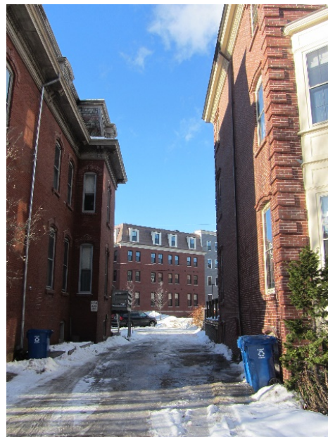
Rear as viewed from Pine St.
