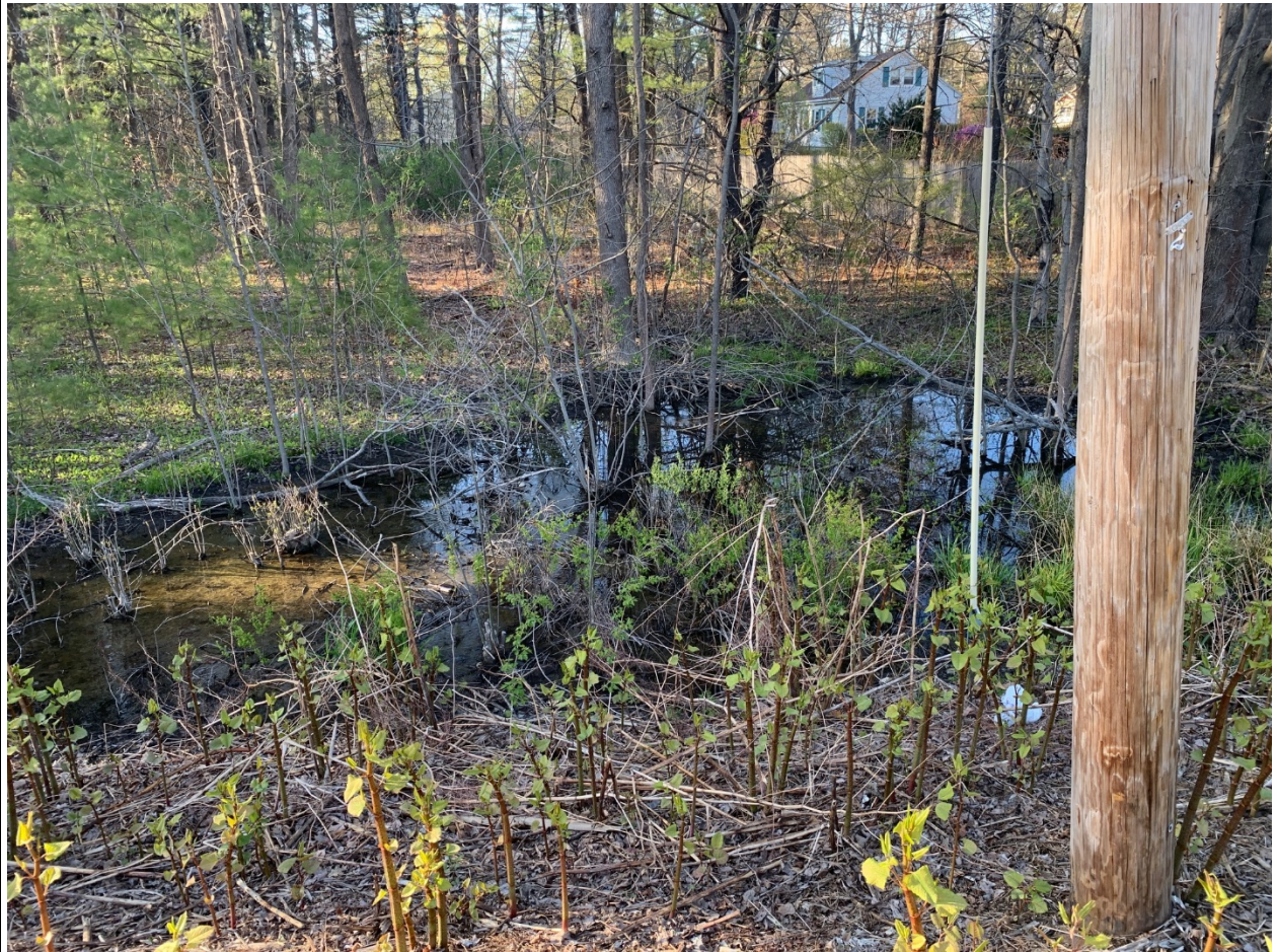
Drainage/Pooling Along Road – May 12, 2020
