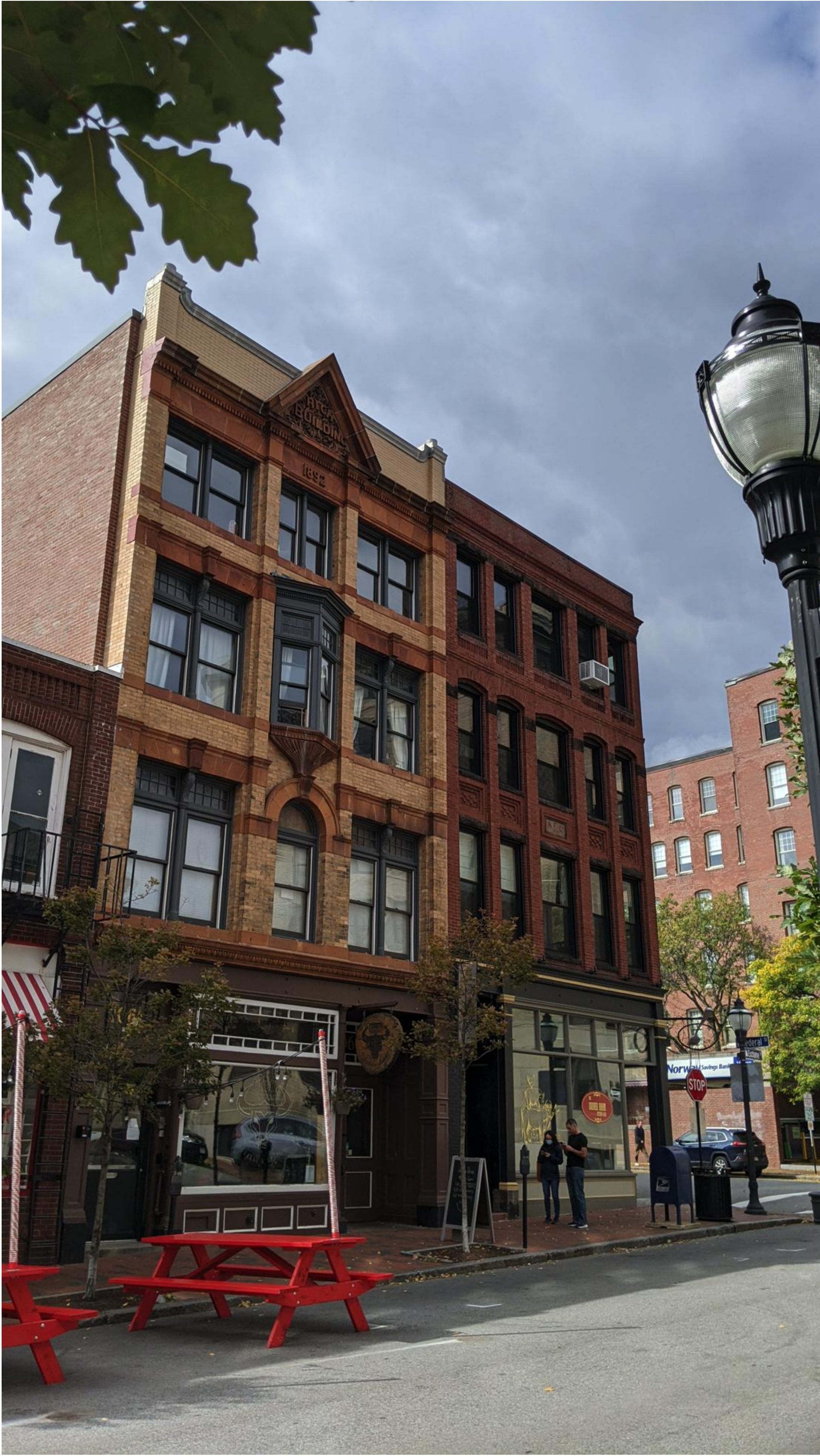
EXISTING - VIEW FROM EXCHANGE LOOKING NORTH
