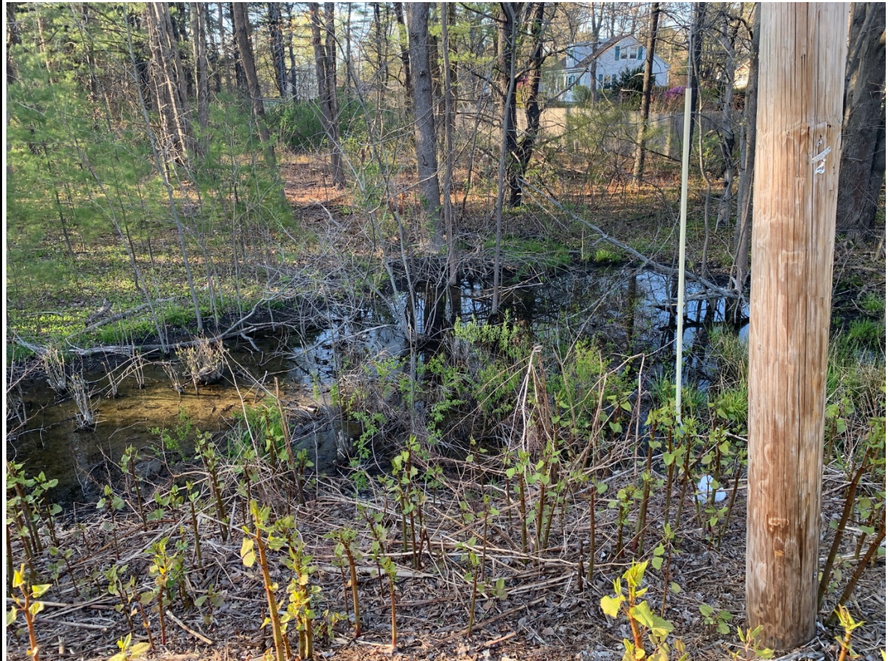
Drainage/Pooling Along Road – May 12, 2020
