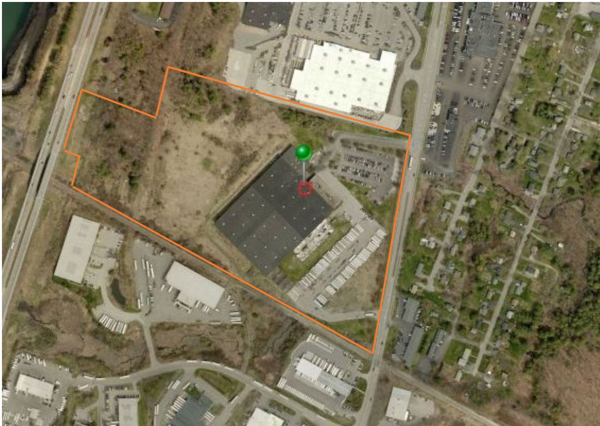
Fig. 1: Surrounding context of 7 Rand Road, highlighted in orange
