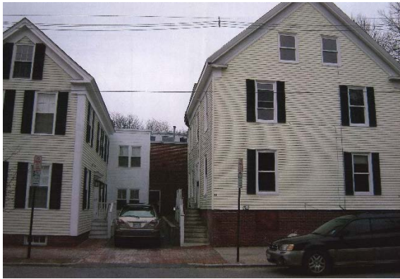
Existing RMDH (left) and abutting house (right) proposed for adaptive reuse and expansion.
