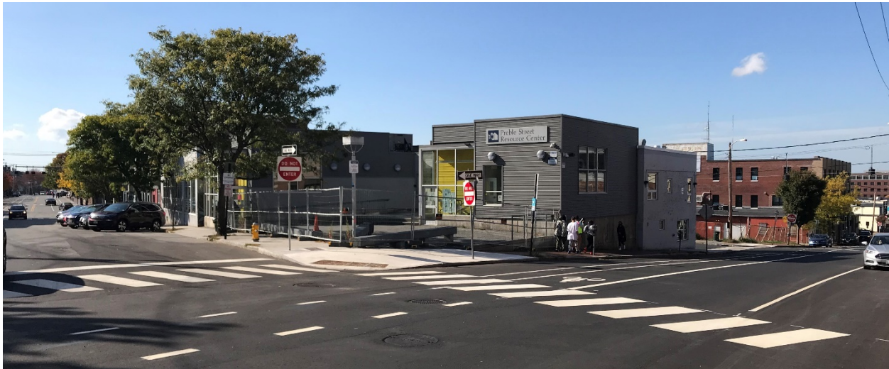
Street View of 5 Portland Street – Source: Andrew Tufts
