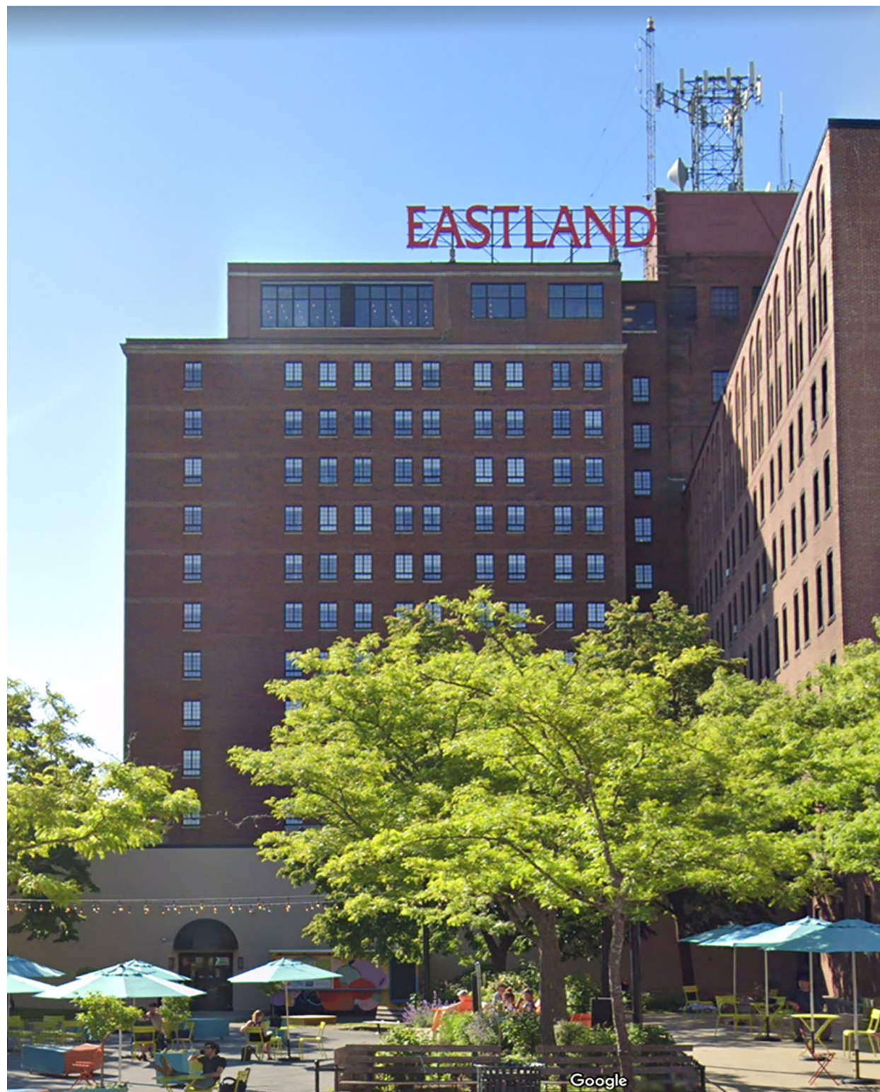
EXISTING - VIEW FROM CONGRESS SQUARE PARK
