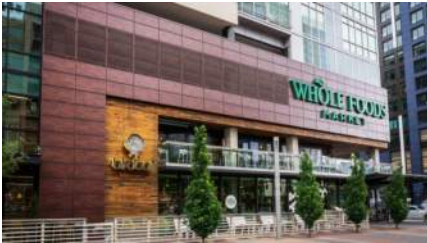
UNION DENVER All Projects, Mixed Use, Wall, Wewatta Rust
