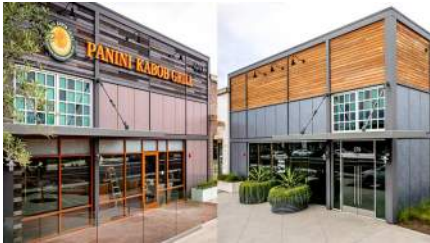
LONG BEACH EXCHANGE All Projects, Blue Rust, Retail, Tempest Patina, Wall
