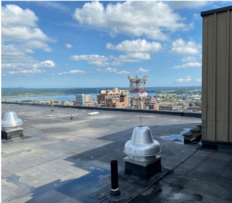
EXISTING ROOF LOOKING NORTHWEST
