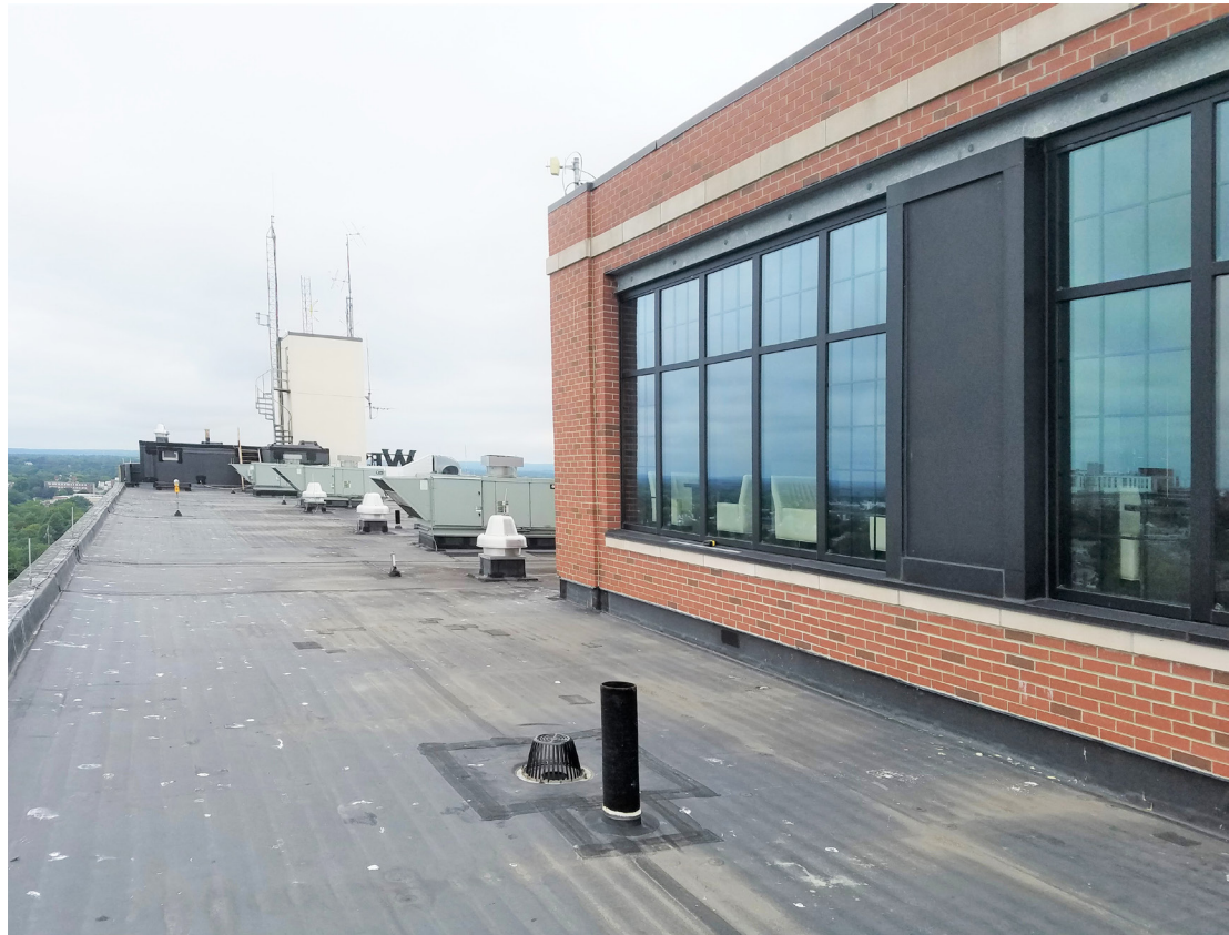
EXISTING 2012 FACADE LOOKING WEST
