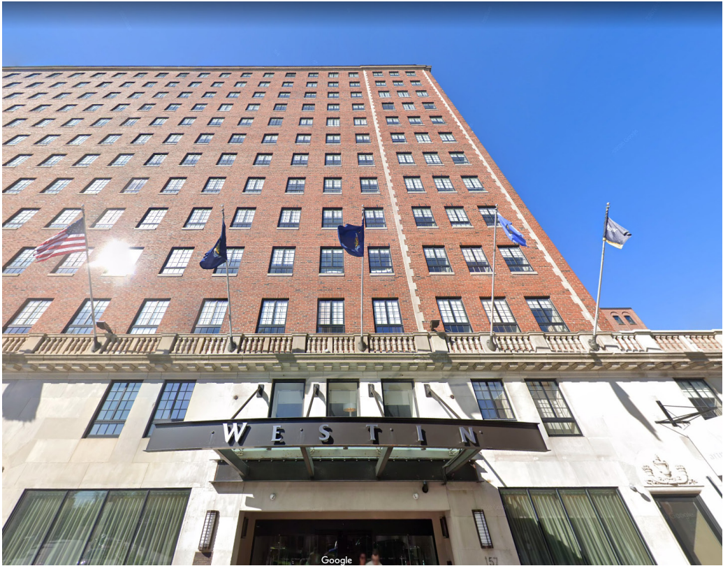
EXISTING VIEW FROM HIGH STREET
