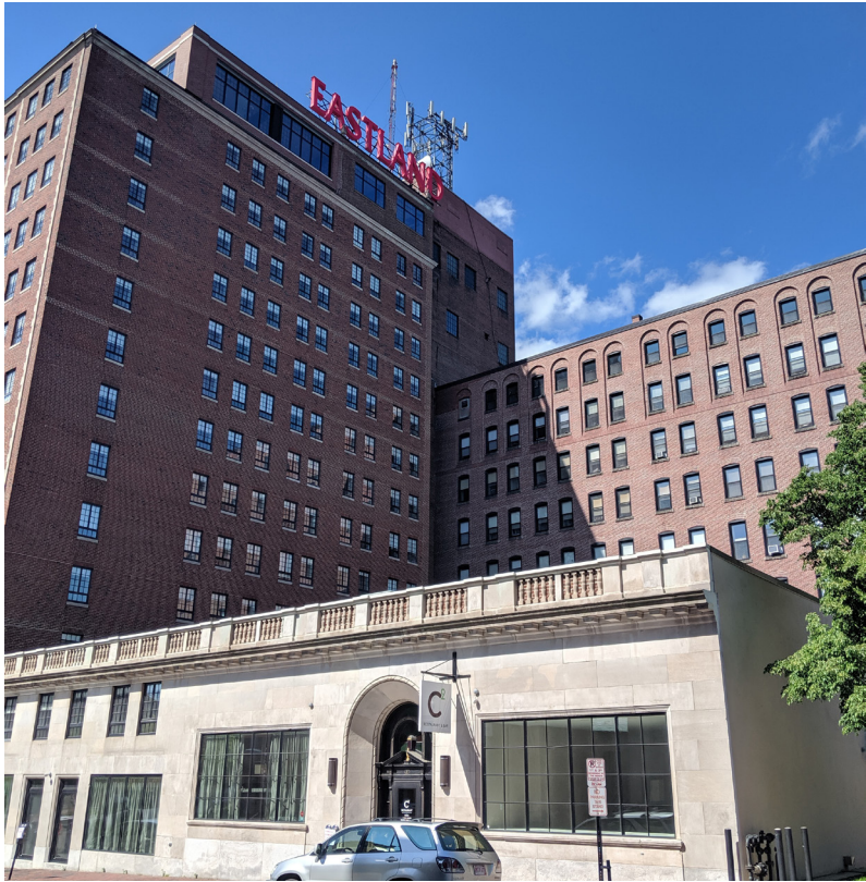
EXISTING VIEW FROM HIGH STREET
