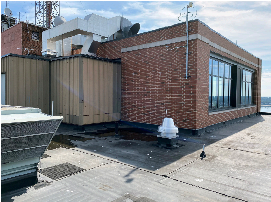
EXISTING EGRESS STAIR PENTHOUSE, MECHANICAL, AND FACADE LOOKING NORTHEAST
