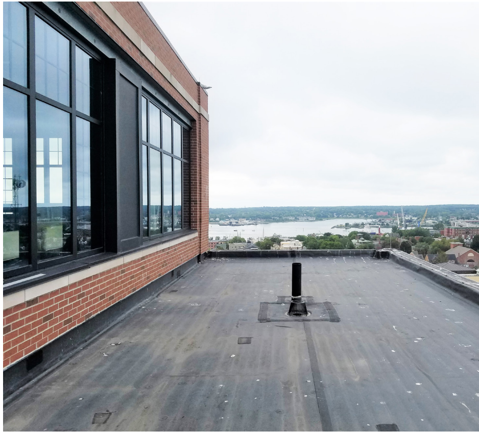
EXISTING 2012 FACADE LOOKING EAST
