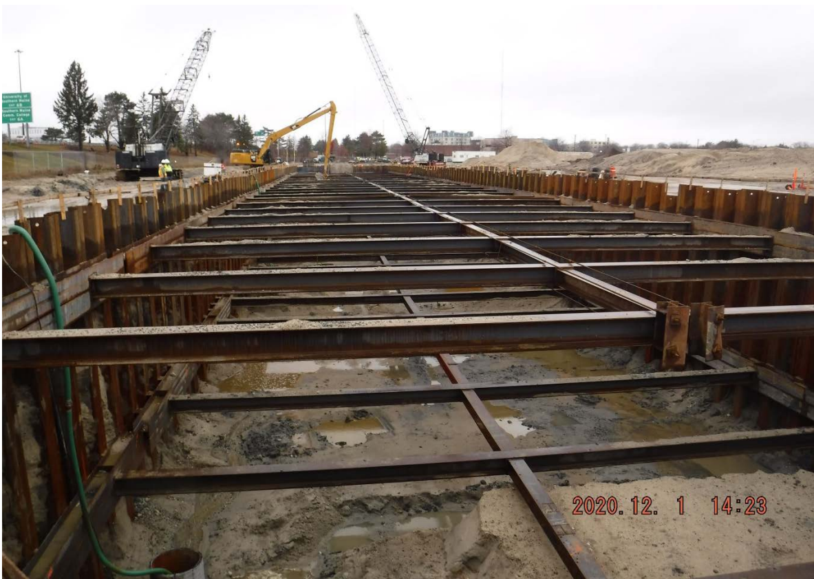
Excavation & bracing on the project site where two of the proposed four storage tanks will be located
