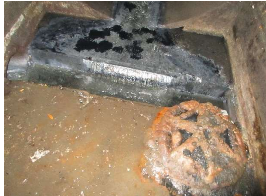
View looking upstream at 72" RC inlet
