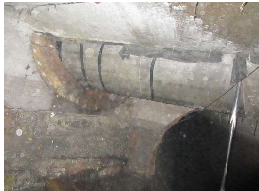
Looking upstream at overhead storm drain
