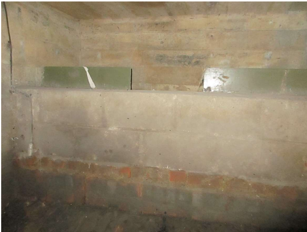
Figure 2-1: CSO 16B Regulator Structure Weir
