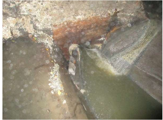
Looking downstream at 36" RC outlet
