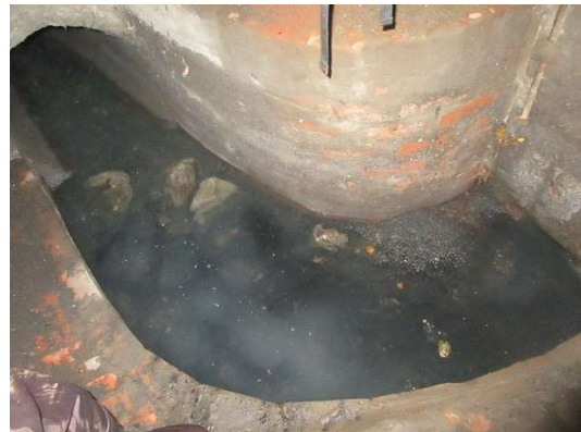
View looking upstream at 24" RCP inlet
