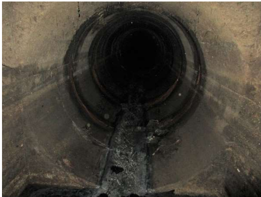
View looking upstream toward 72" RC inlet
