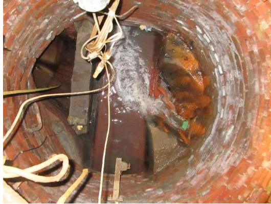
View looking down into brick manhole
