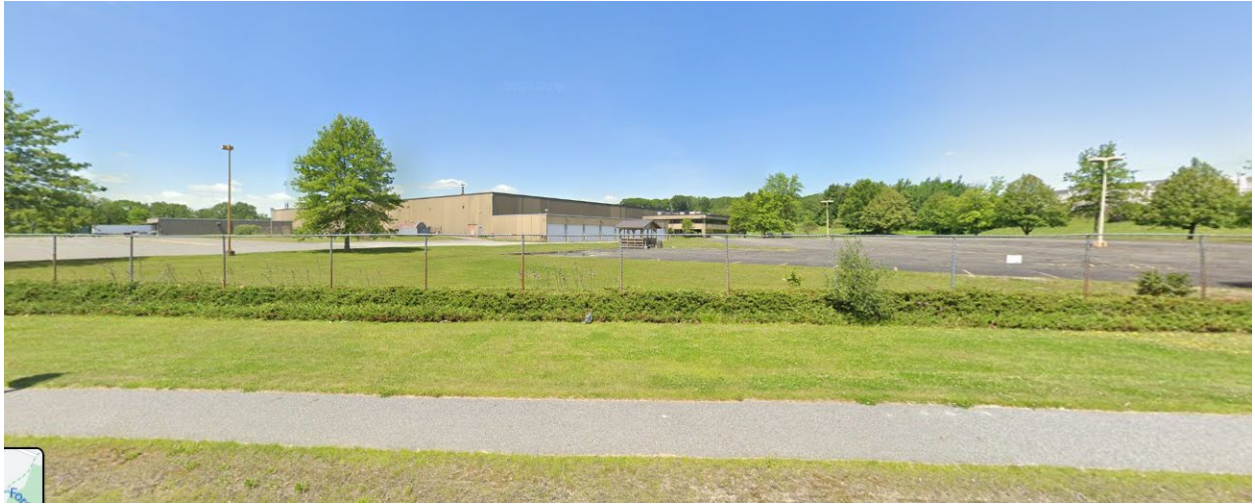
Fig. 4: View of subject property from Rand Road
