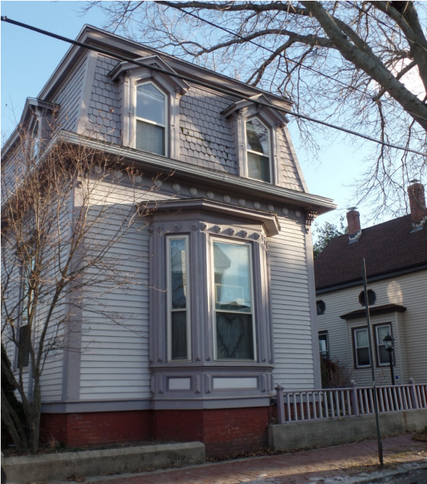
The Alfred Roberts House (1876) at 80 Quebec Street.
