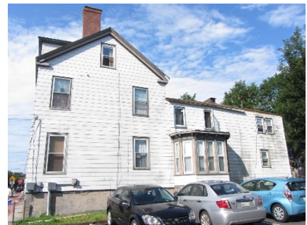
Approval rec'd to demolish ell.
