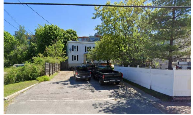
Figure 3: Street Level View of Existing Property
