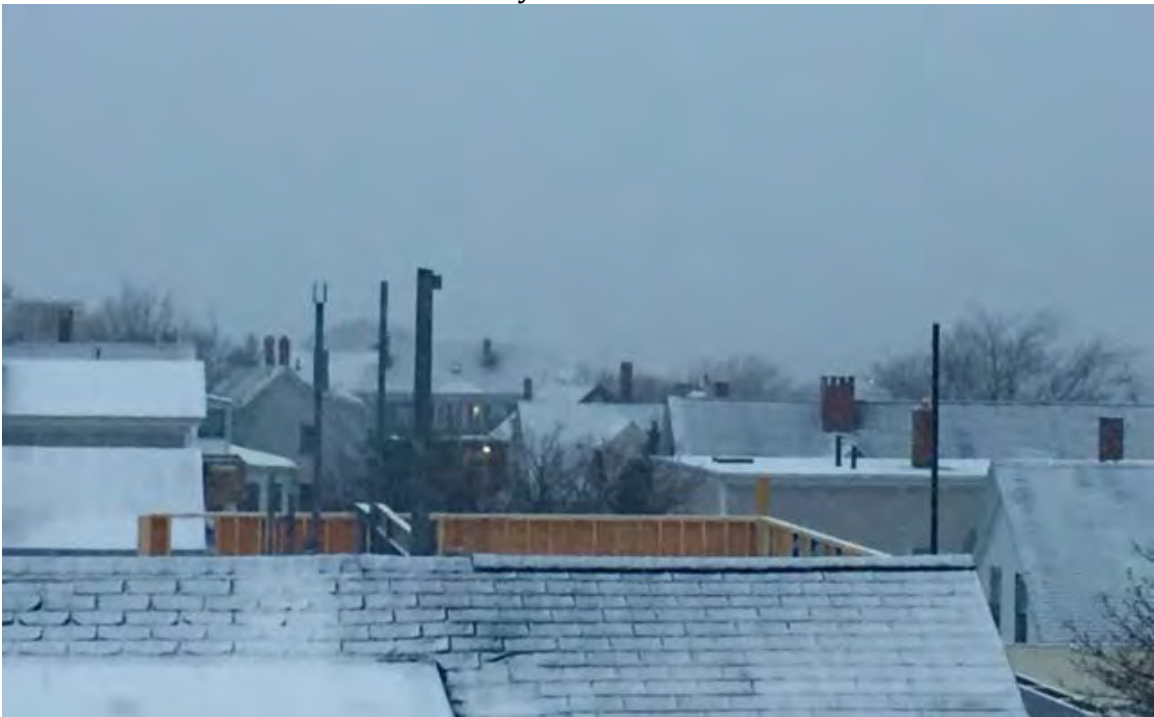
12.28.18 New Construction at 9 Moody Street
