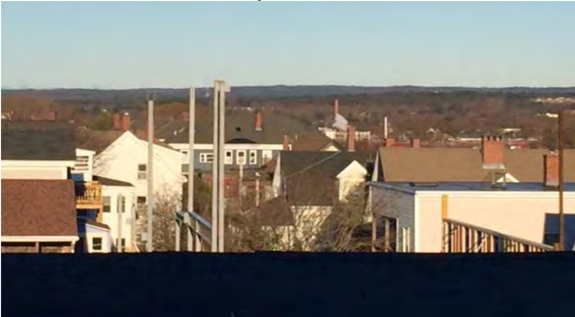
12.23.18 New Construction at 9 Moody Street
