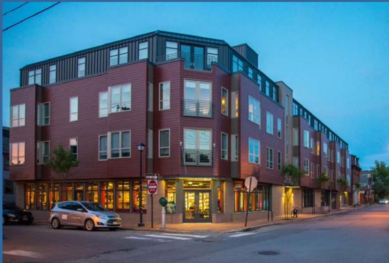
Solar panels cover the roof of this new construction project in the West End Historic District
